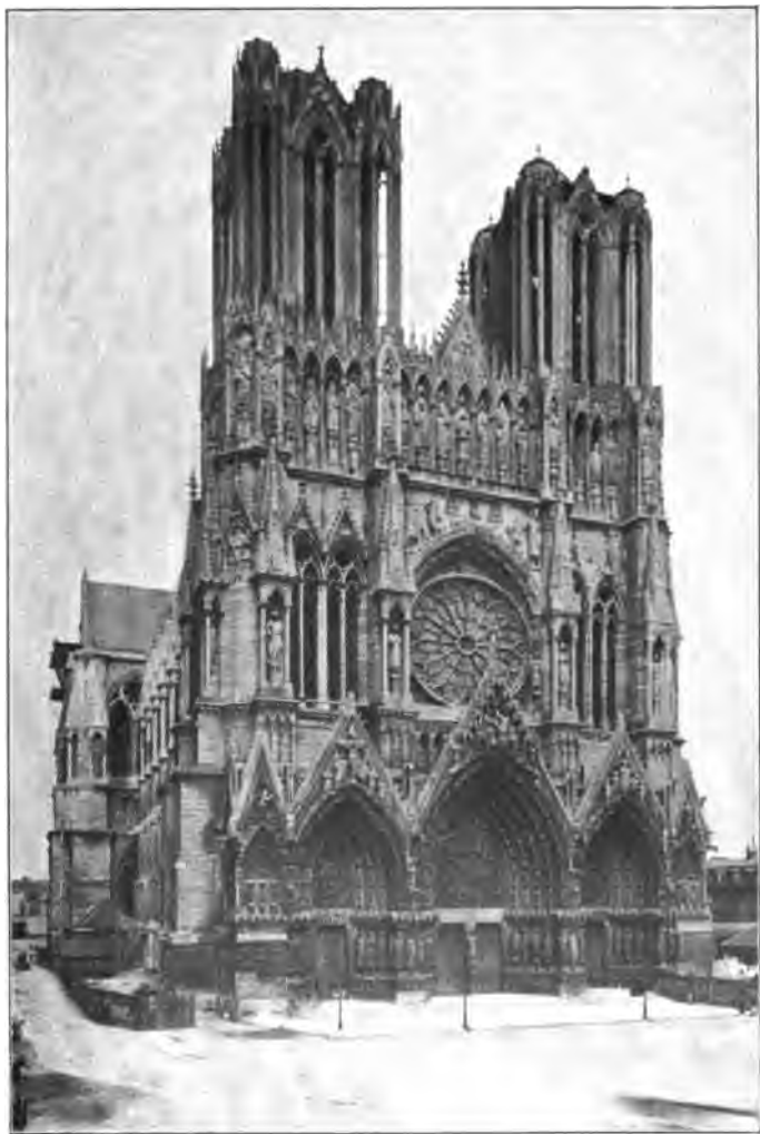
FAÇADE OF RHEIMS CATHEDRAL
