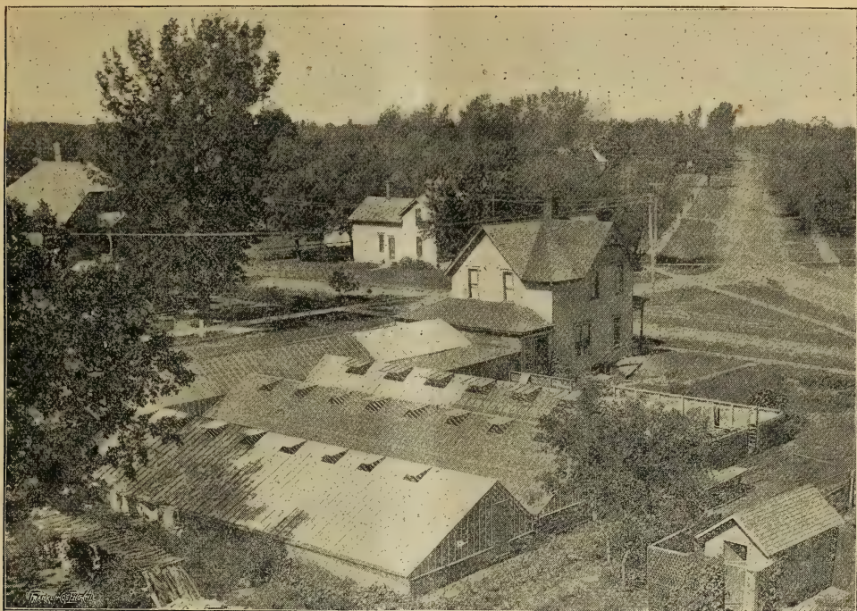
Austin Green Houses. (From a Photograph.)
