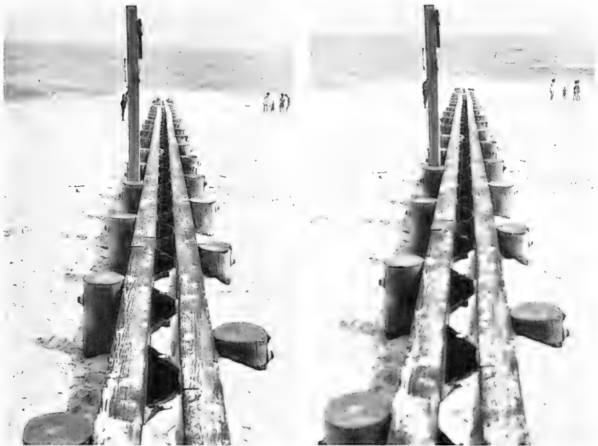
FIGURE 5. COMPARATIVE PHOTOS DOWN THE AXIS OF A GROIN. THE PHOTO ON THE RIGHT WAS MADE WITH THE FOCUS AT INFINITY; ON LEFT, 30 FEET.
