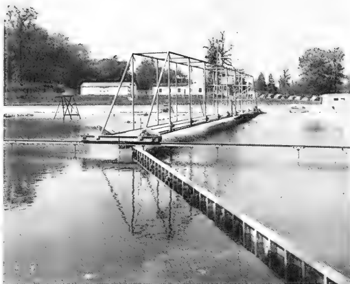
FIGURE 10. INSTRUMENT AND PERSONNEL CARRIER IN THE SHORE PROCESSES TEST BASIN
