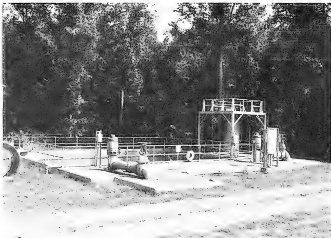
FIGURE 11. TIDE SUMP AND PART OF THE PUMPING SYSTEM FOR THE SHORE PROCESSES TEST BASIN
