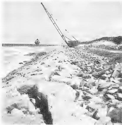
FIGURE 9. STONE REVETMENT - FORT STORY, VIRGINIA
