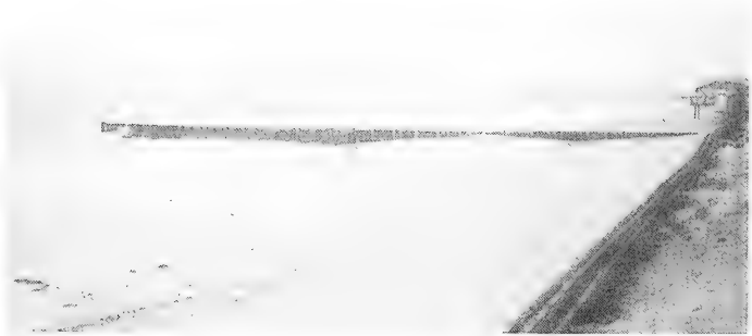
FIGURE 8. TIMBER BULKHEAD AND GROINS - LONG BRANCH, NEW JERSEY
