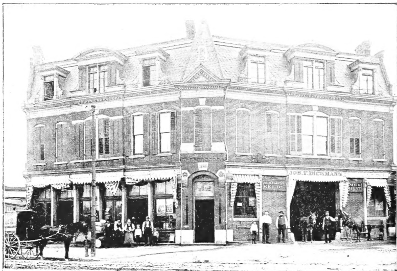
Warehouse and Store, Gravois and Oregon Avenues.
