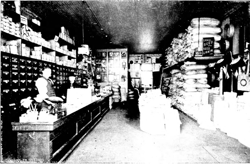
Interior View of Salesroom, 1110 North Third Street.
