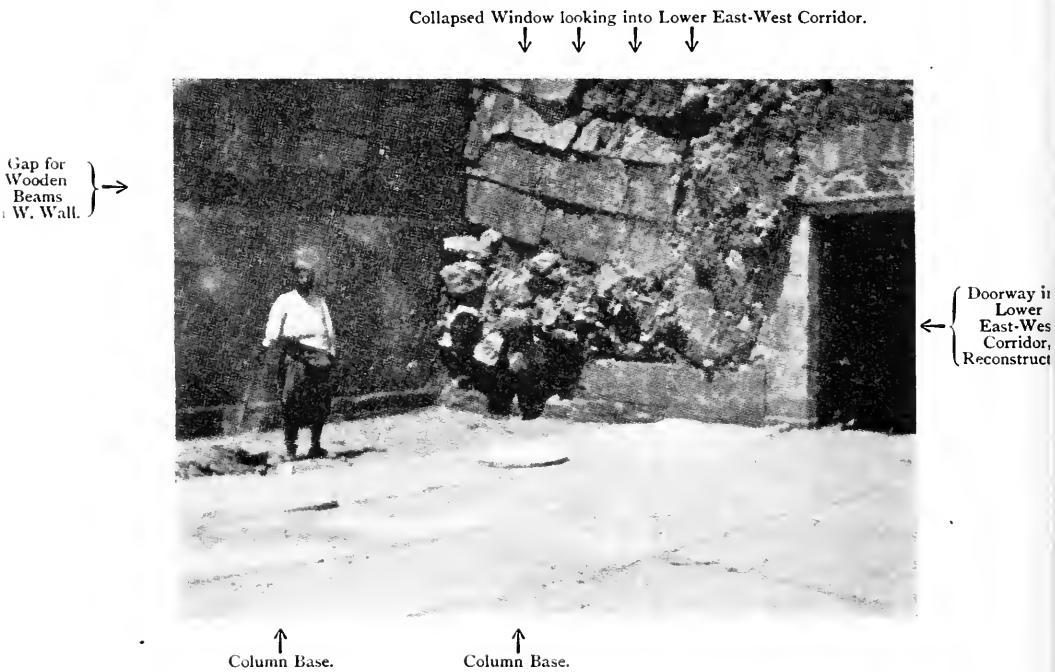
FIG. 21.—VIEW IN HALL OF DOUBLE AXES SHOWING COLLAPSED WINDOW OFF LIGHT AREA.
