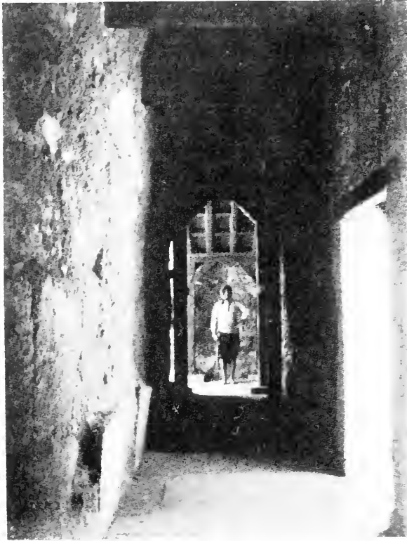
FIG. 16.—VIEW IN LOWER EAST-WEST CORRIDOR (LOOKING E.).
