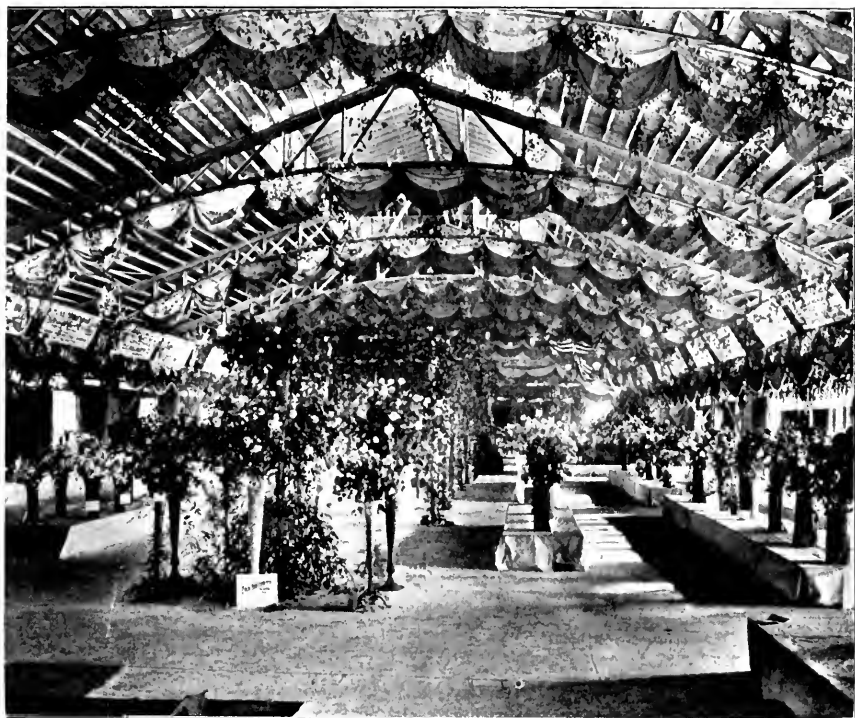
ONE VIEW OF THE 1912 EXHIBITION, LOOKING THE LENGTH OF THE BUILDING.
