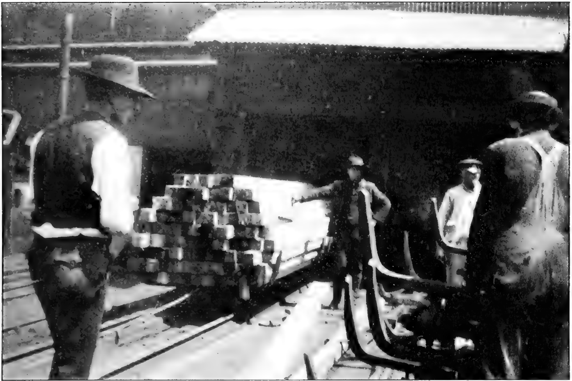
CAR LOADED WITH TIMBER ( 3\frac{3}{4} \times 4 SEWER STAVES) ENTERING CYLINDER.
