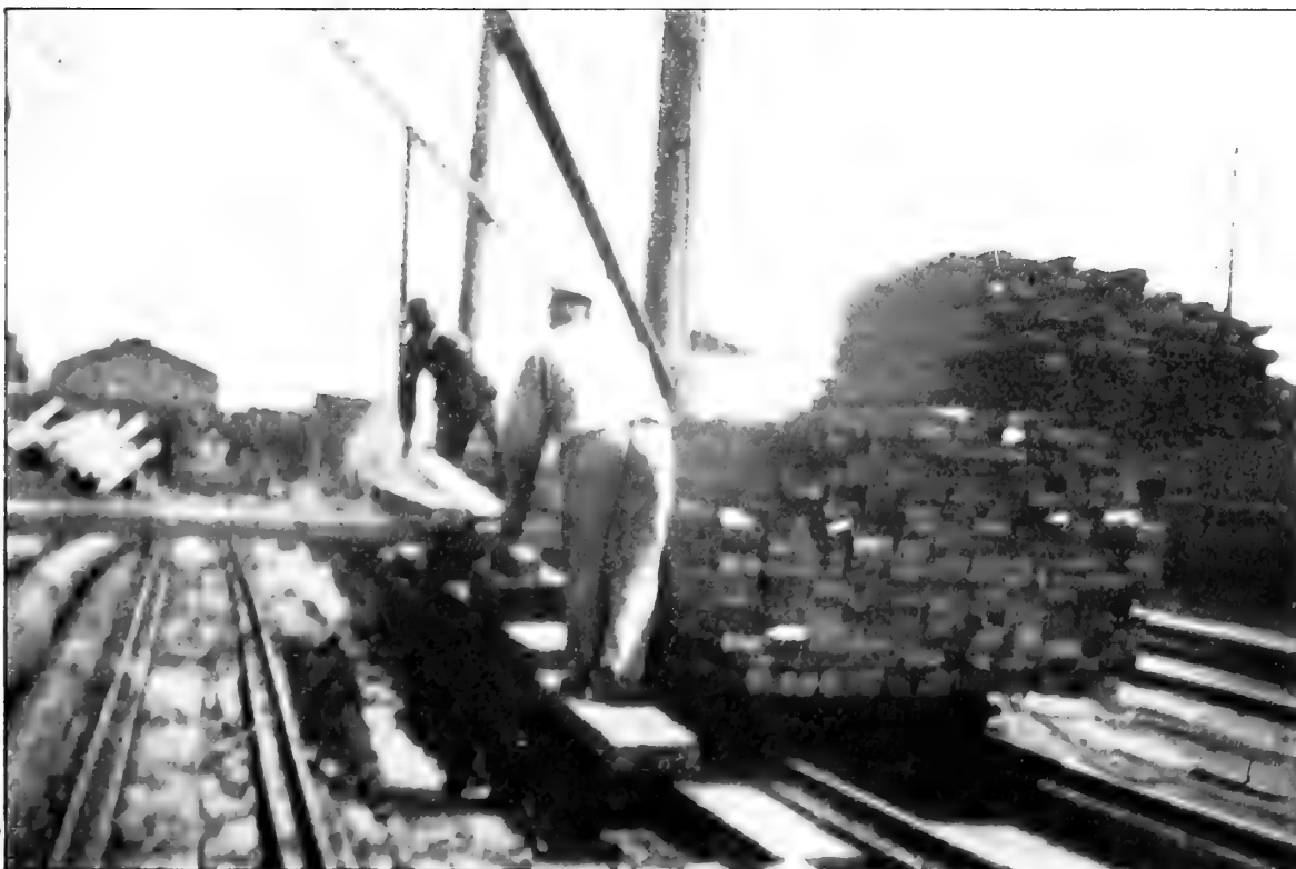
UNLOADING 2 X 6 TONGUE-AND-GROOVE PLANKS, WHICH HAVE JUST BEEN TREATED.
