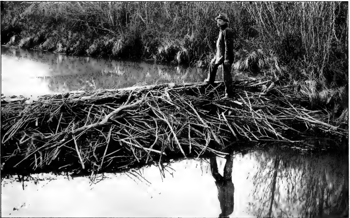
DAM CONSTRUCTED OF LARGER STICKS.
