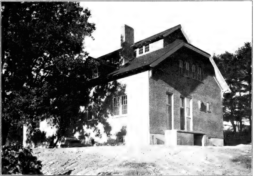
Fruit Storage Building and Laboratory, erected in 1910-11.
