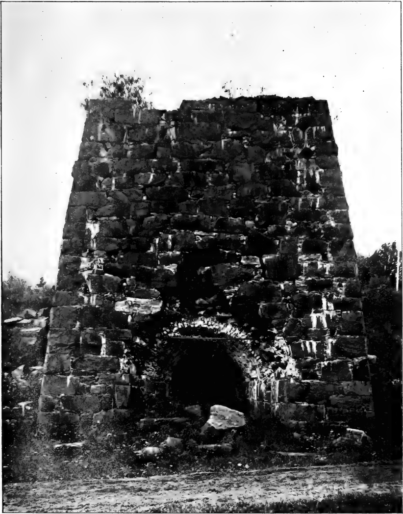
Colburn furnace, a charcoal stack built in 1848, about 1 mile west of Moriah Center, near Mineville
