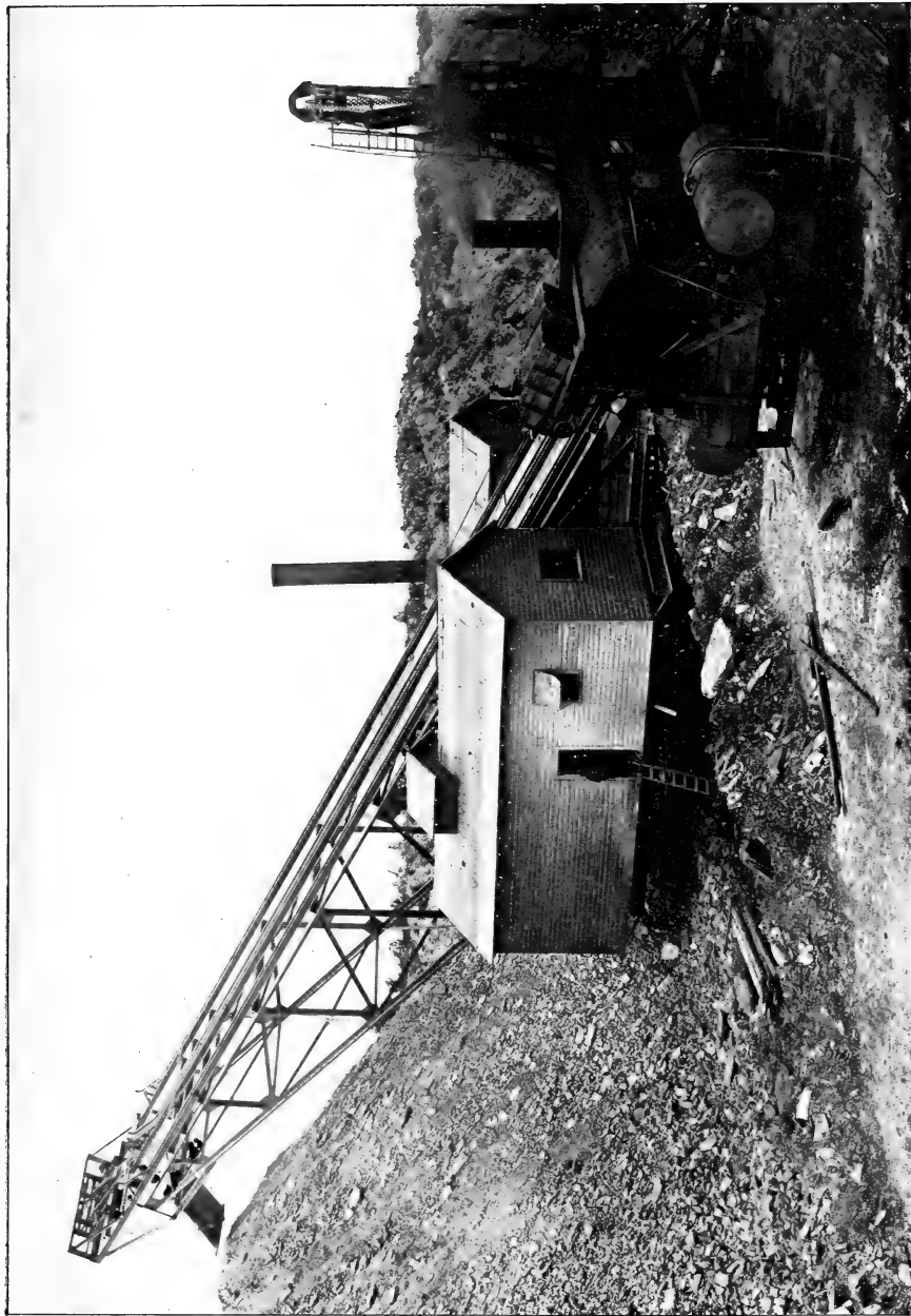
View showing steam shovel and conveyor used to remove the overburden from the ore. Furnaceville Iron Co., Ontario Center, Wayne co.
