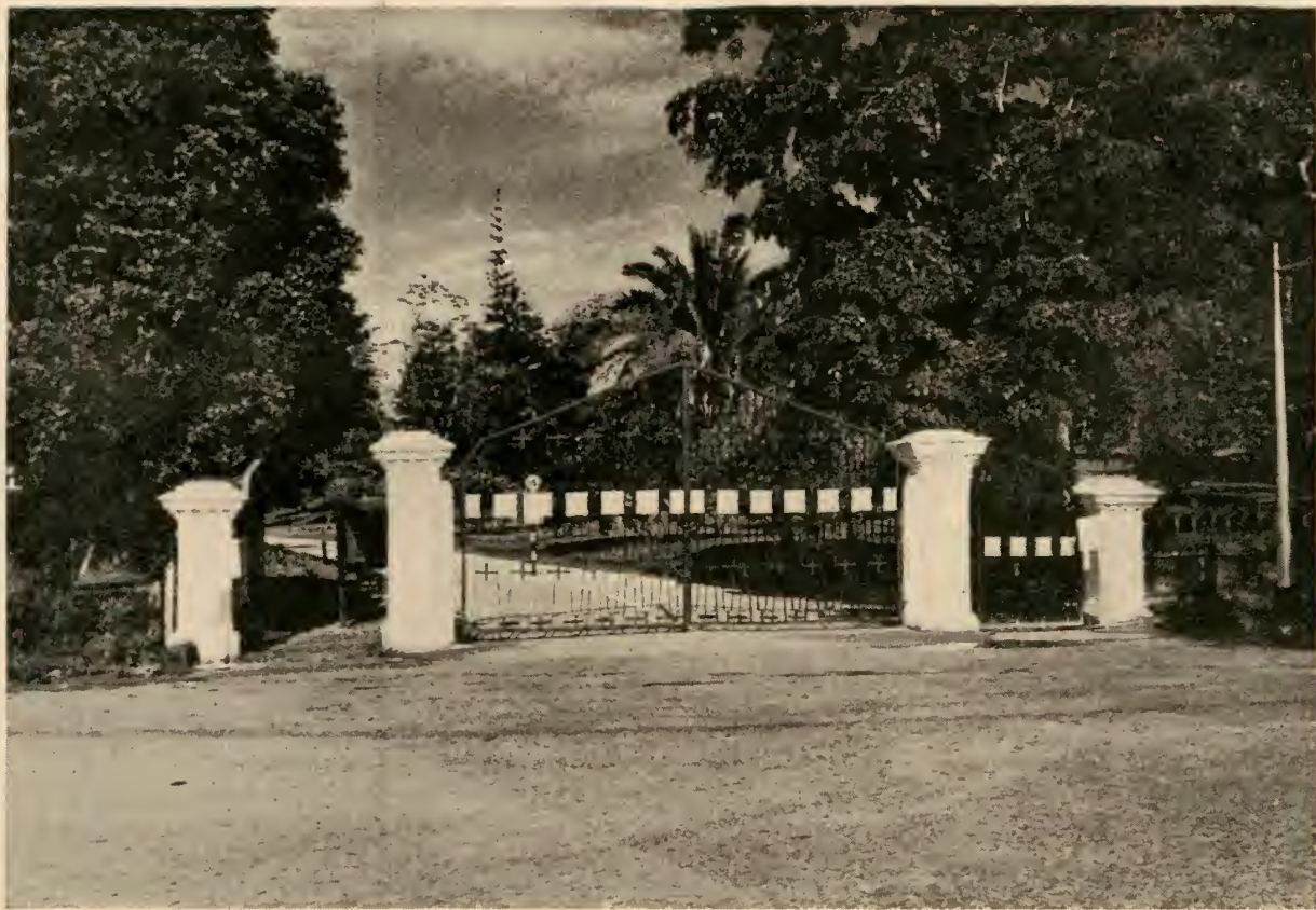
Plate 1. New Gates erected January 1964: one pair road gates and two side pedestrian gates
