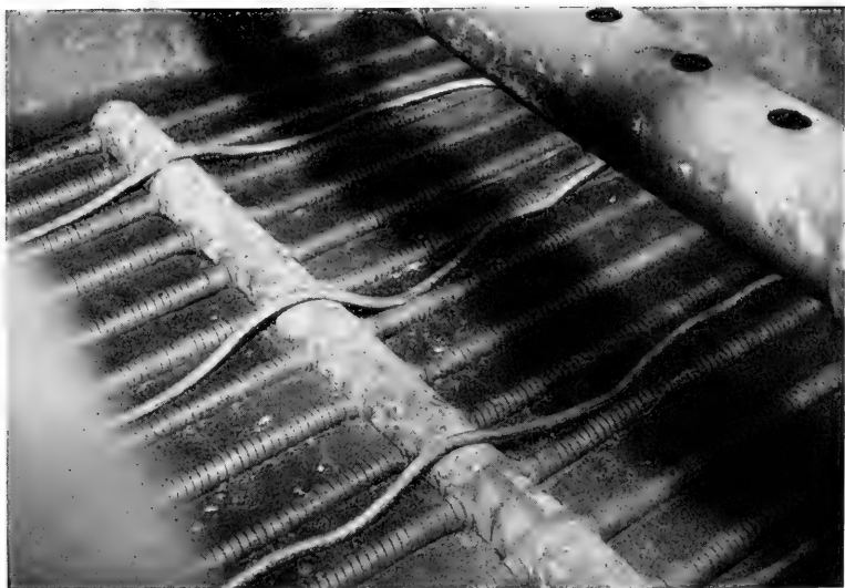
FILTER BED OF LEAD PIPES HALF-BEDDED IN CEMENT, THE EXPOSED SURFACES HAVING INNUMERABLE, FINE CROSSWISE SAW CUTS TO SECURE RAPID DRAINAGE
