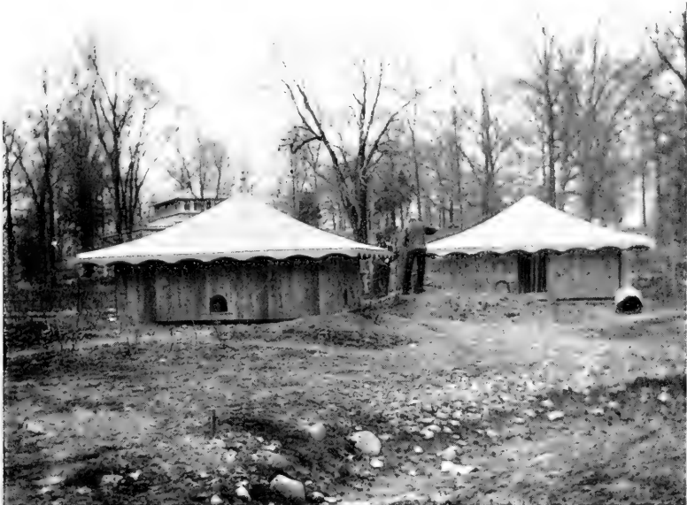
ERECTING DUCKS' SHELTER HOUSES.
