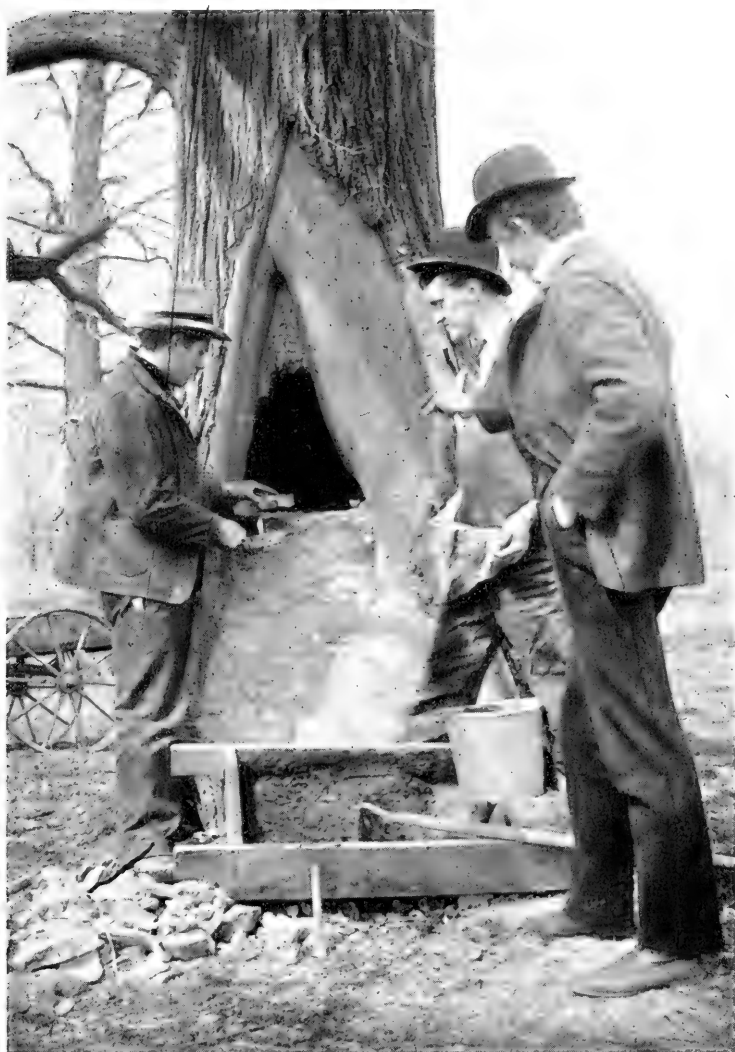
REPAIRING FIRE DAMAGES, WITH MASONRY.
