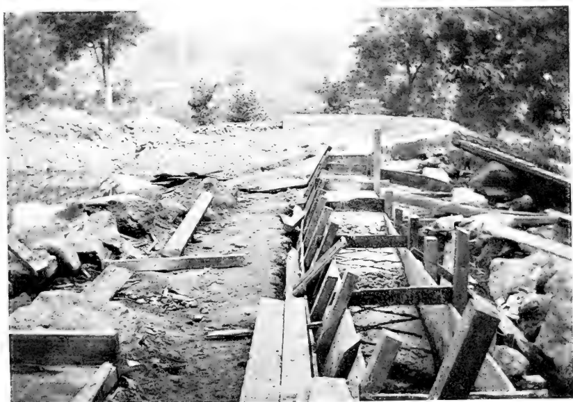
BUILDING CONCRETE COPING AT WATERFALL.
