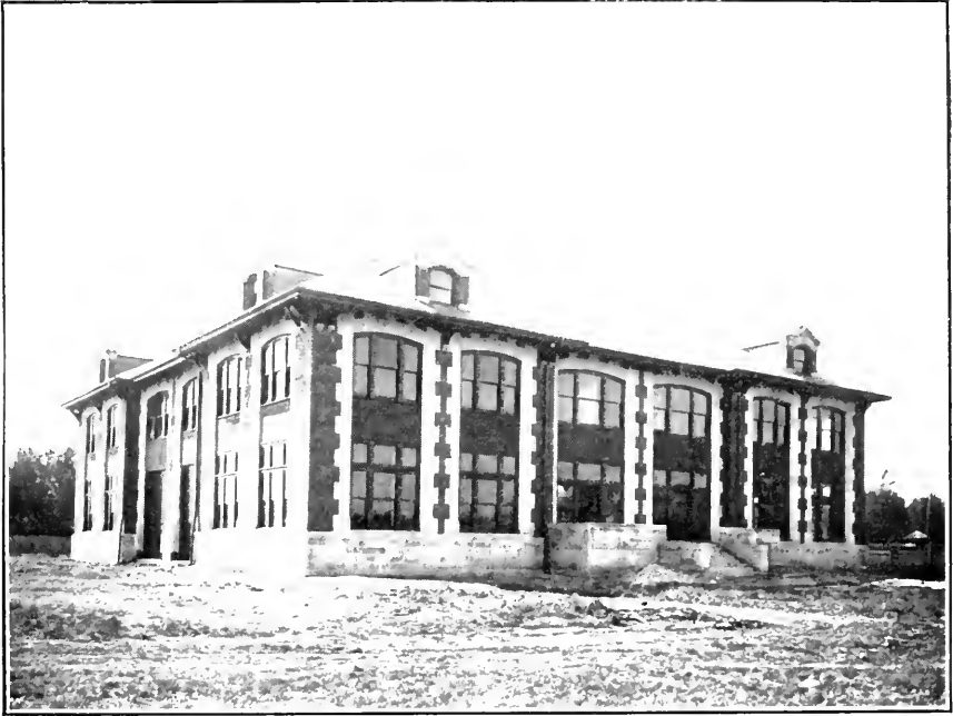
FIG. 1.—NEW FARM MECHANICS BUILDING, UNIVERSITY OF ILLINOIS.
