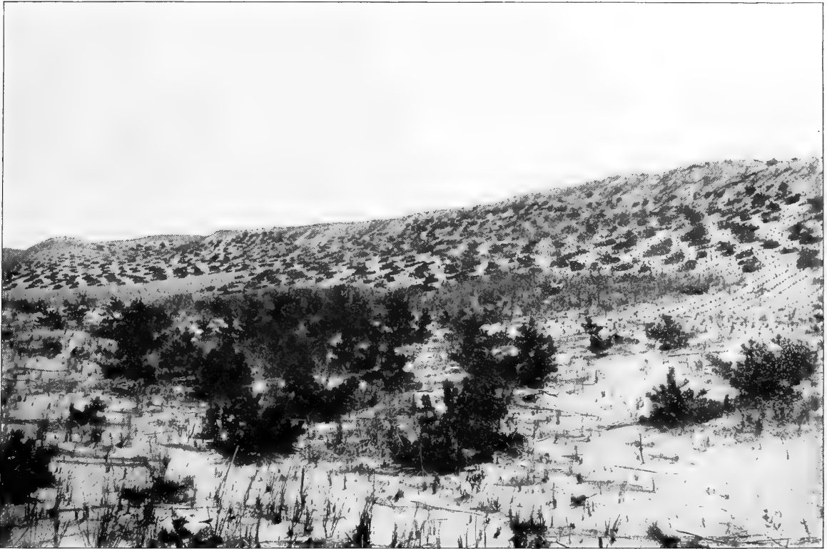
No. 1.—PLANTATION OF BEACH-GRASS AND PITCH-PINE ON CAPE COD, FOR THE FIXATION OF THE SOIL.
