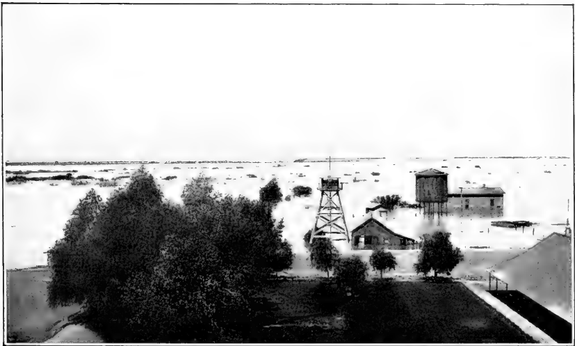
LOOKING SOUTHERLY OVER TEMPORARY DIKES IN THE SUBMERGED TOWNS OF CALEXICO AND MEXICALA.
