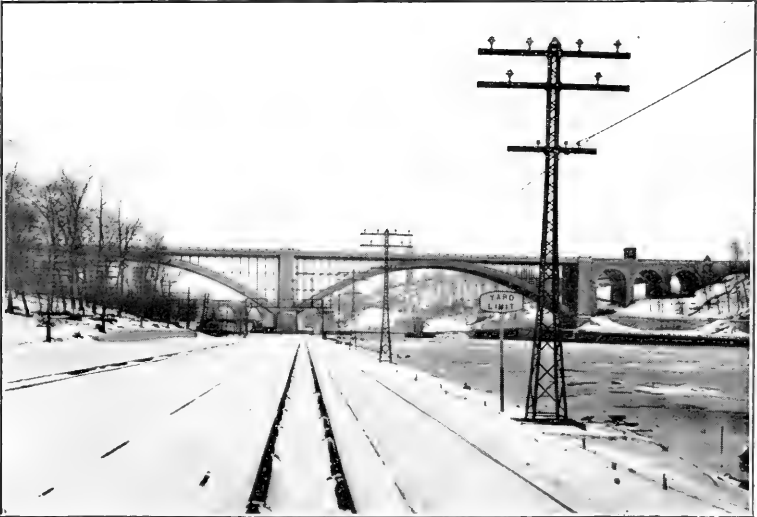
PROTECTED THIRD RAIL BURIED IN SNOW.
