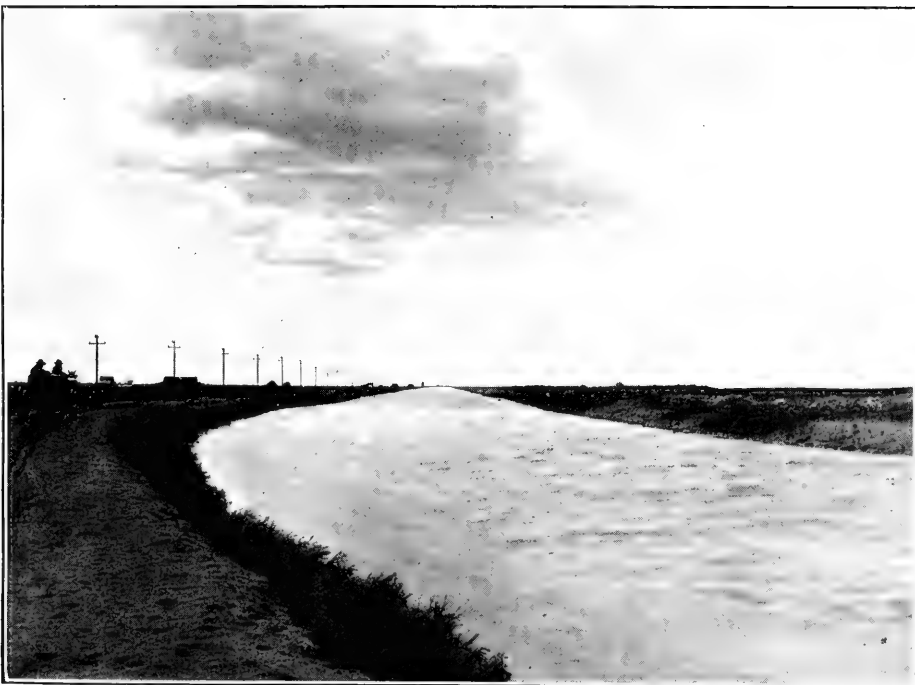
2. MAIN NORTHSIDE CANAL, MINIDOKA PROJECT, IDAHO, TYPICAL OF THE LARGER IRRIGATION CANALS, WITH POWER TRANSMISSION LINES LOCATED ON THE BANK.
