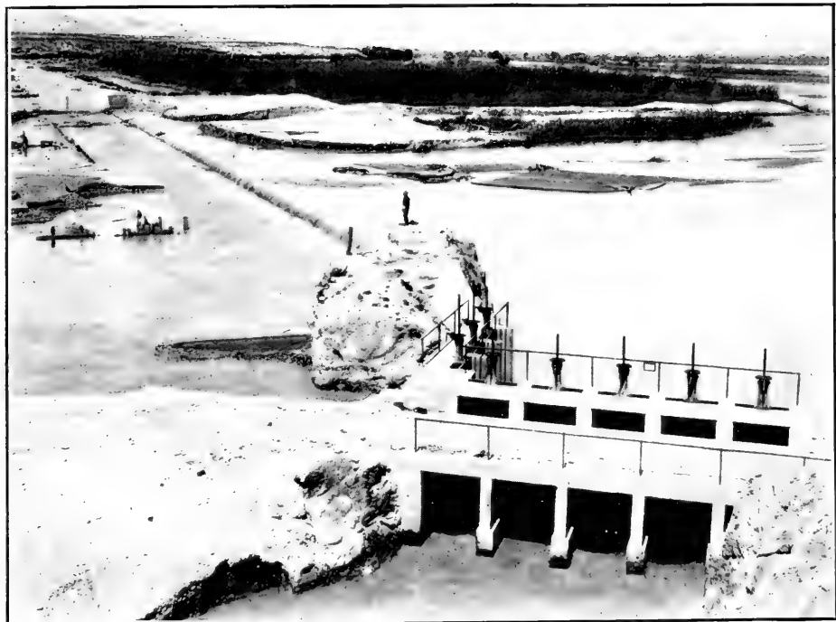
2. DIVERSION DAM AT LEASBURG, NEW MEXICO, ON RIO GRANDE, AND HEAD OF CANAL FOR MESSILLA VALLEY.
