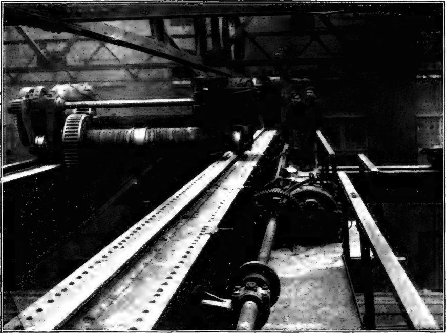
1. ELECTRIC TRAVELING CRANE BOUGHT ABOUT TEN YEARS AGO.
