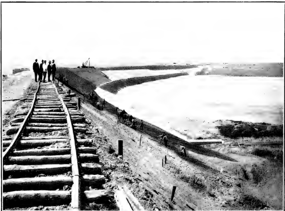
2. EARTHEN DAM FOR OWL CREEK RESERVOIR, BELLE FOURCHE PROJECT, SOUTH DAKOTA.
