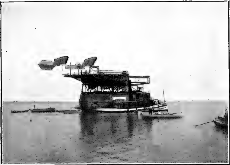
1. HOUSE-BOAT AND LAUNCHING APPARATUS FOR LANGLEY AERODROME, 1899.
