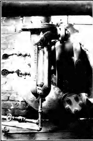
1. GAUGE GLASS FOR INDICATING HEIGHT OF WATER IN A BOILER. SEMICIRCULAR STEEL GUARD SHOWN IN ITS NORMAL POSITION.
