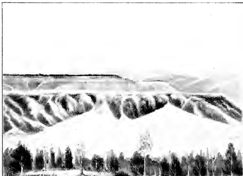
EFFECT OF HYDRAULIC SLUICING OF UPPER WHITE GRAVELS, BONANZA CREEK, KLONDIKE.
