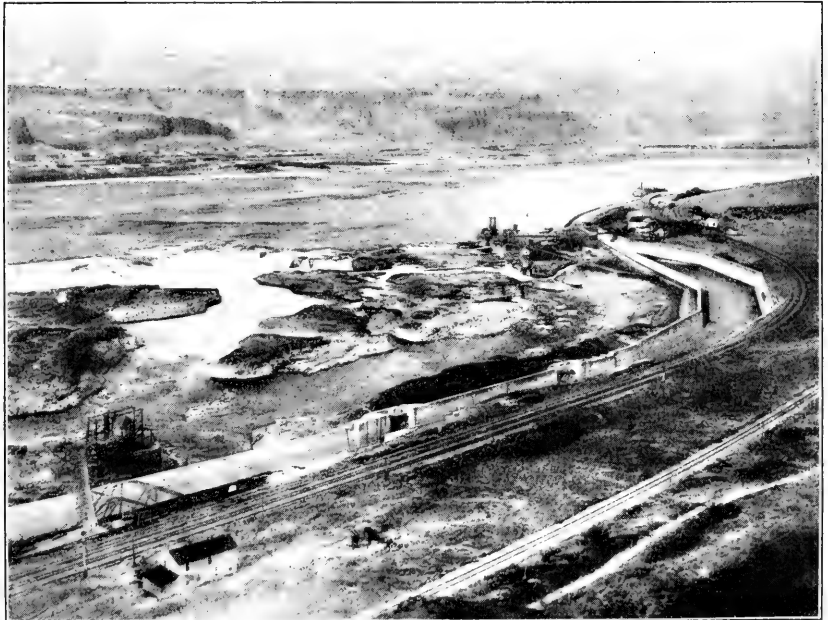
2. THE UPPER END OF THE DALLES-CELILO CANAL, COLUMBIA RIVER, OREG. SIDE WALLS OF CONCRETE CARRY THE CANAL TRUNK AROUND CELILO FALLS.
