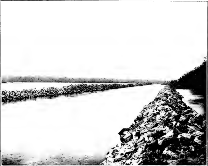
1. A ROCK CUT ON THE TENNESSEE RIVER SHOWING TRAINING WALLS ALONG THE SIDES, AND A CONTRACTING SPUR ON THE LEFT.
