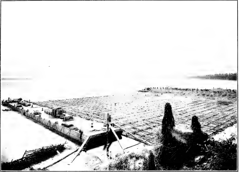
1. MAT WOVEN OF POLES AND BRUSH FOR BANK PROTECTION ON THE MISSISSIPPI RIVER. THIS MATTRESS IS CONTINUOUS, AND IS BUILT ON THE SCOW SHOWN ON THE RIGHT.
