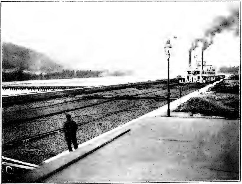
2. A FLEET OF COAL BARGES PASSING LOCK NO. 2, OHIO RIVER. THE MOVABLE DAM IS UP AND IS SHOWN ON THE LEFT.
