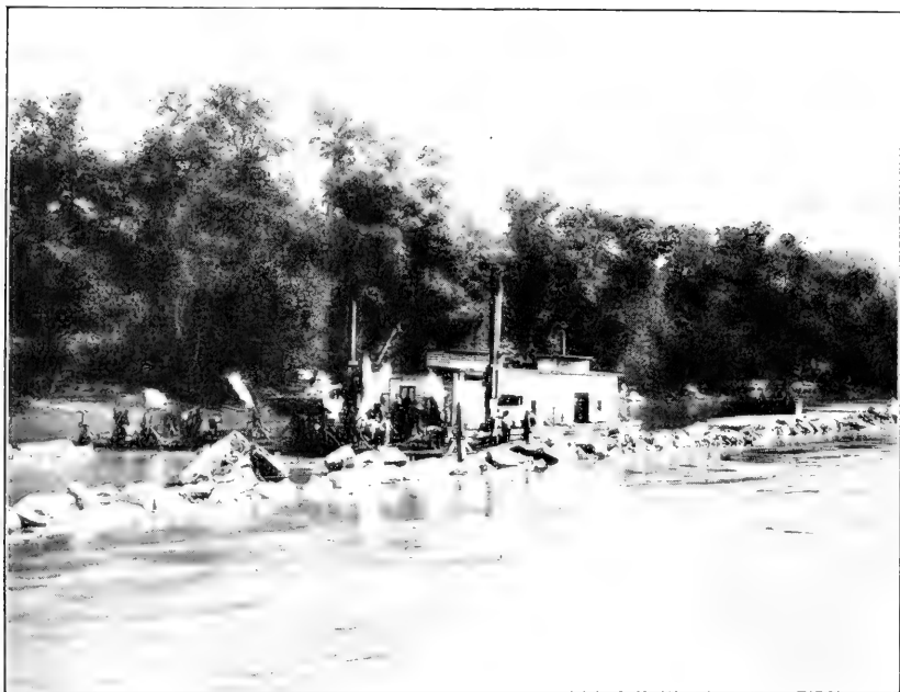
1. ROCK EXCAVATION ON THE TENNESSEE RIVER. SPECIALLY DESIGNED DRILL RAFT BORING PREPARATORY TO BLASTING.
