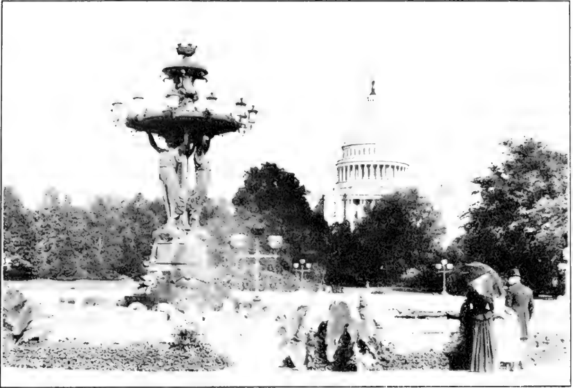
1. The Capitol on the middle Columbian terrace as seen in 1890 from the Bartholdi Fountain on the lower one.
