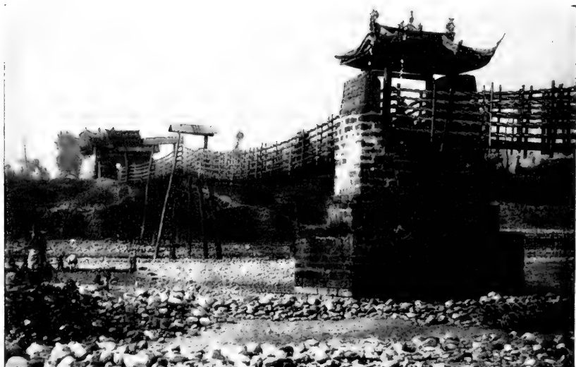
2. CHINESE SUSPENSION BRIDGE WITH BAMBOO CABLES.
