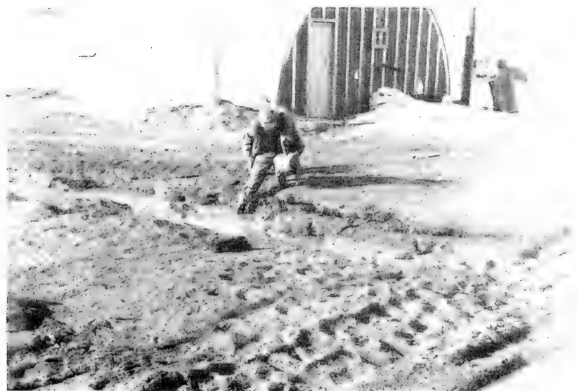
2. Slump in gravel on street in Barrow, where steam line produced thawing of permafrost. Photographed May 12, 1950.
