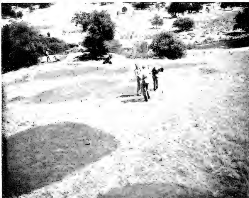
2. Starting excavations at the Terminus Reservoir in California. The locations of the house pits are shown by the dark circles on the surface of the ground.
