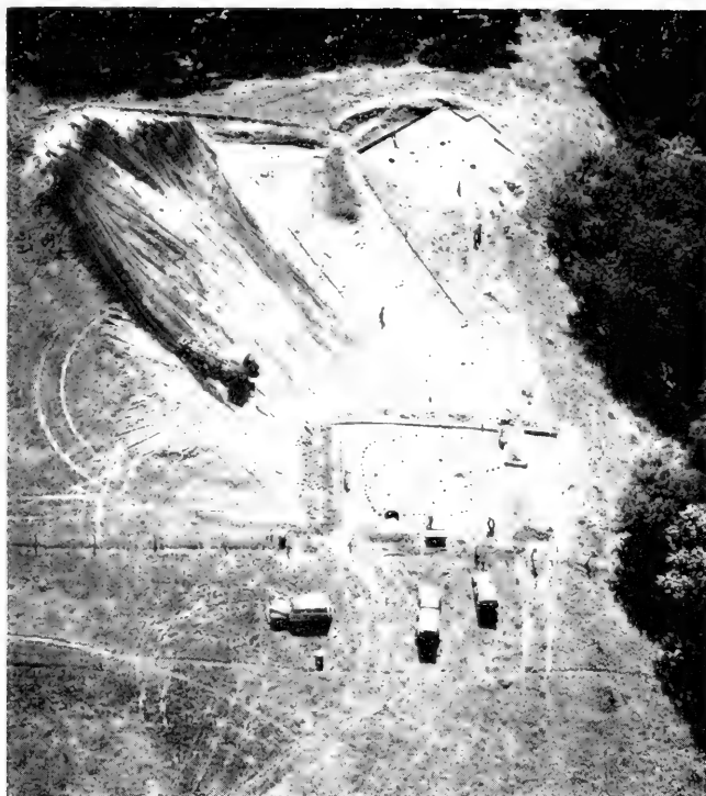
1. Uncovering house floors at the Medicine Creek Reservoir in western Nebraska. The highway patrol, which was used to strip off the overburden, may be seen to the left of the lower house.
