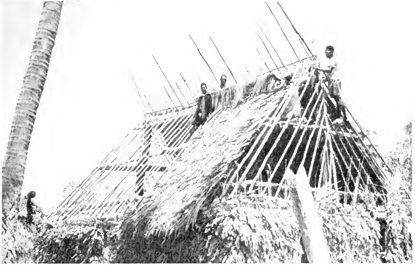
1. The frame of the roof of a new house is made of saplings lashed together, and on this the Metroxylon "shingles" are tied with fibers.
