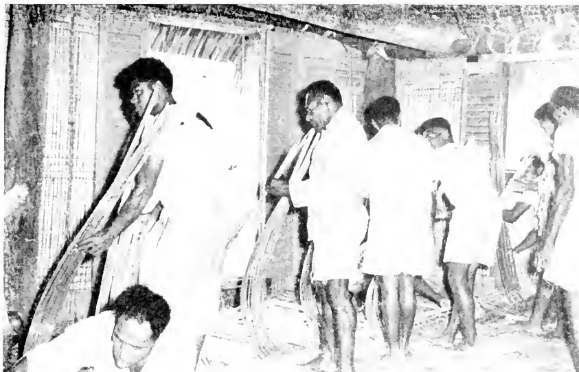
1. An introduced bamboo, Bambusa vulgaris , is widely utilized. Here a floor of woven split bamboo is being laid in a new house. The reeds lining the walls, of the large grass Miscanthus japonicus , are woven together with coconut or hibiscus fibers. Many species of forest trees produce the huge timbers that Fijians use in their houses, which are built entirely without the use of metal fastenings.
