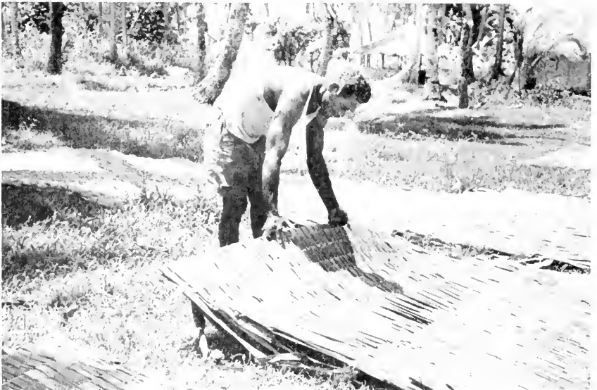
2. The leaf segments of Metroxylon vitense are taken from the leaves, bent around a reed, and sewed together with hibiscus fiber. "Shingles" about six feet long are dried in the sun and then tied to the rafters of the roof. Such thatching is said to be durable for 20 years or more.
