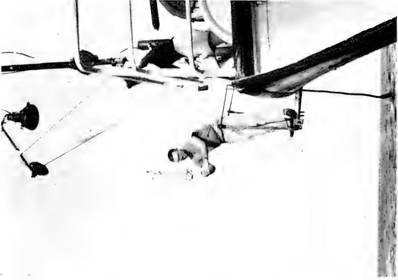
2. Working water-sampling bottles from the forecastle head of the Discovery II .
