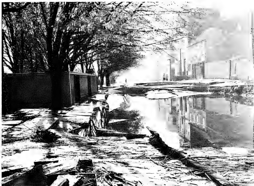
1. Damage to Malecón and park in Valdivia resulting from failure of retaining wall and artificial fill.
