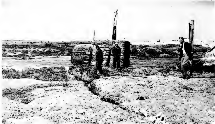
1. Dock at Isla Mocha destroyed by tsunami and former shoreline raised 2\frac{1}{2} meters. Before, top of concrete was awash at low tide. Picture taken at high tide.
