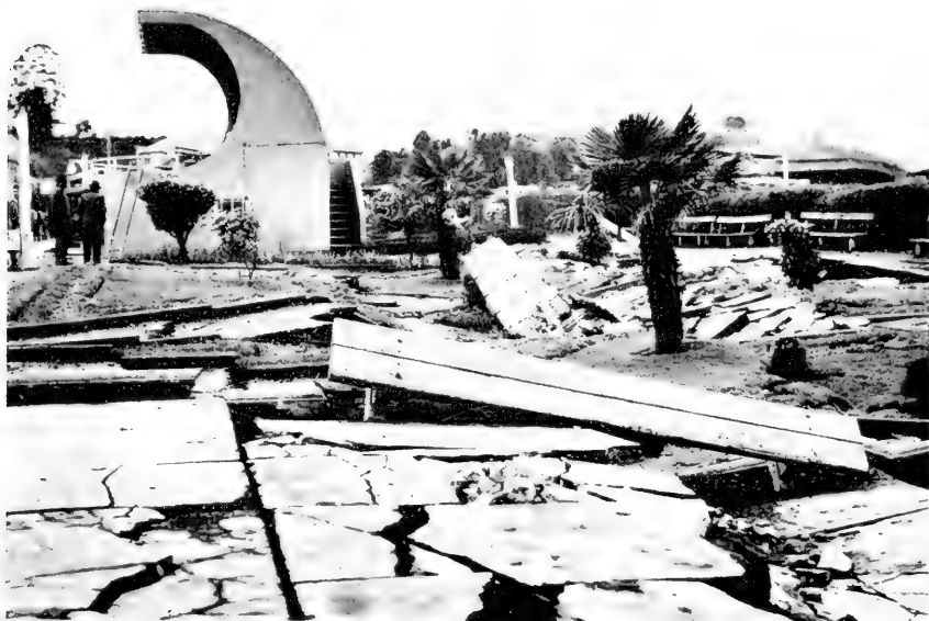
2. The public square in Puerto Montt. Liquefied soil caused the statue to sink.
