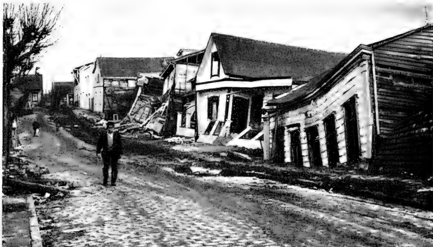
1. Damage to good-quality, wood-frame houses in Valdivia caused by solifluction and sliding of the houses toward a small, now abandoned stream channel to the right.
