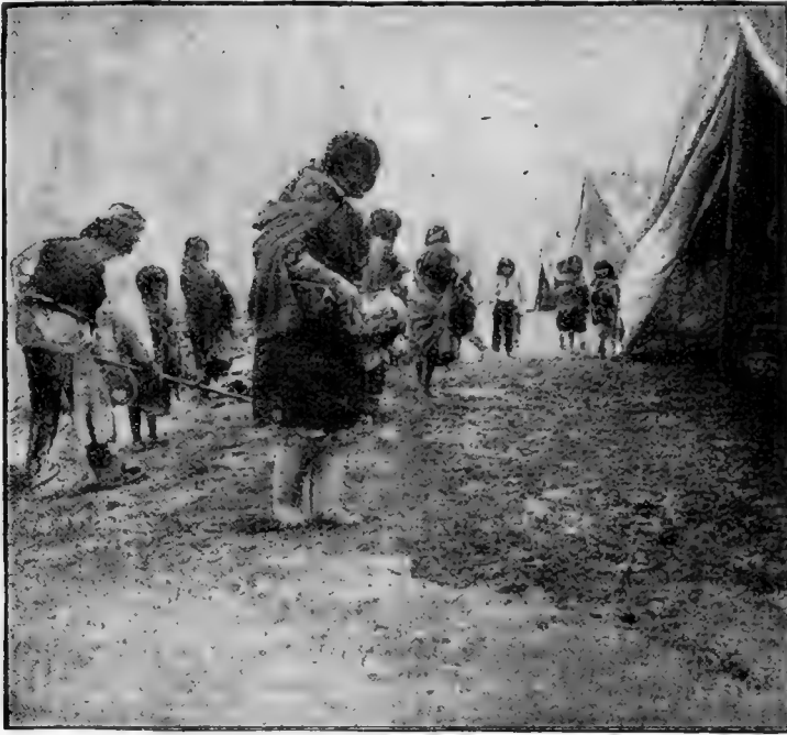
FIG. 10.—The process of leveling.
