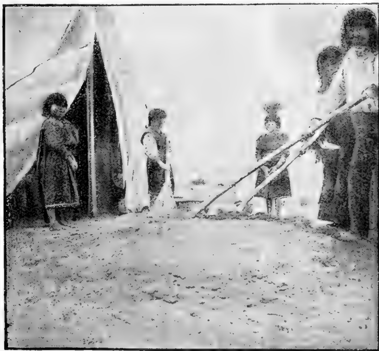
FIG. 12.—Mixing clay for plaster.
