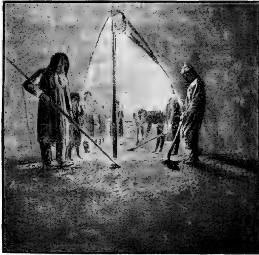
FIG. 4.—Breaking the earth under tent.
