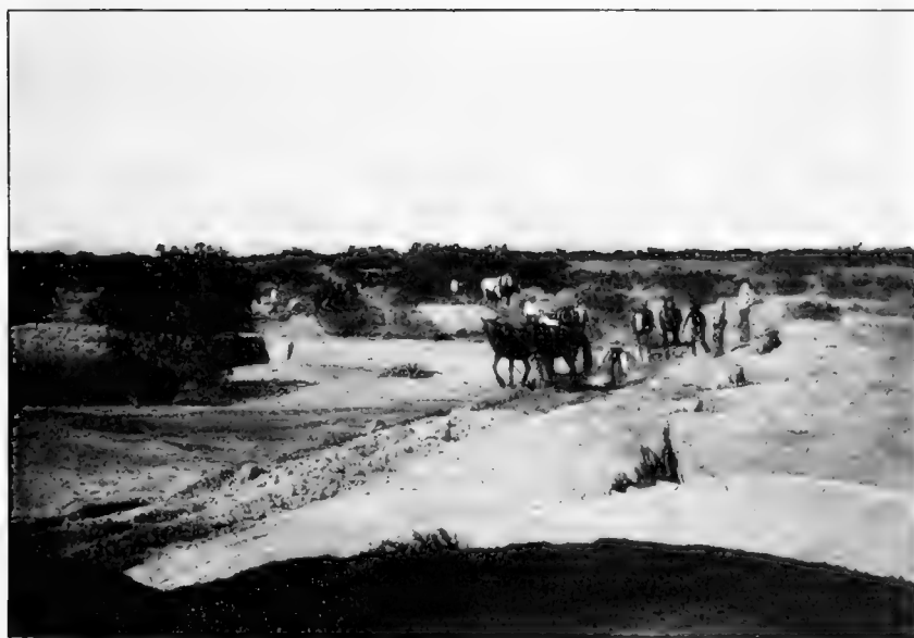
NORTHWEST PLAZA, EAST SIDE, SHOWING WORK OF EXCAVATION CEREMONIAL ROOMS AND PLAZA, COMPOUND A
