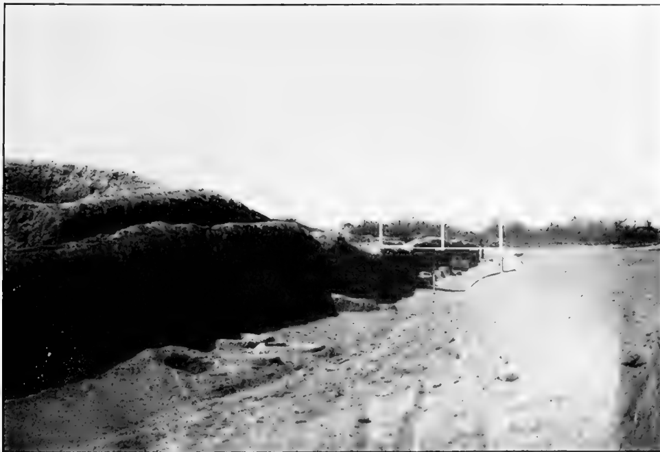
a , WEST WALL. LOOKING SOUTH
