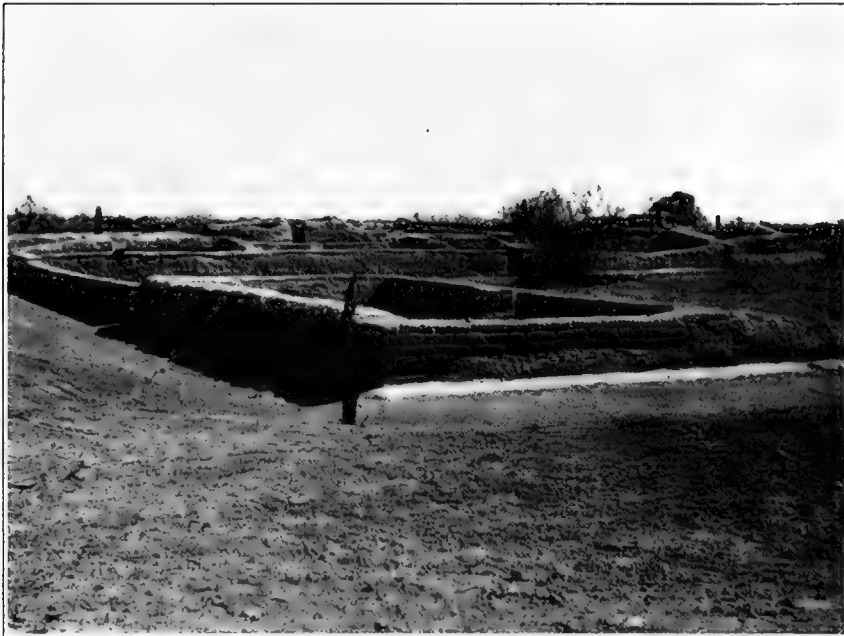
b , NORTHWEST CORNER
