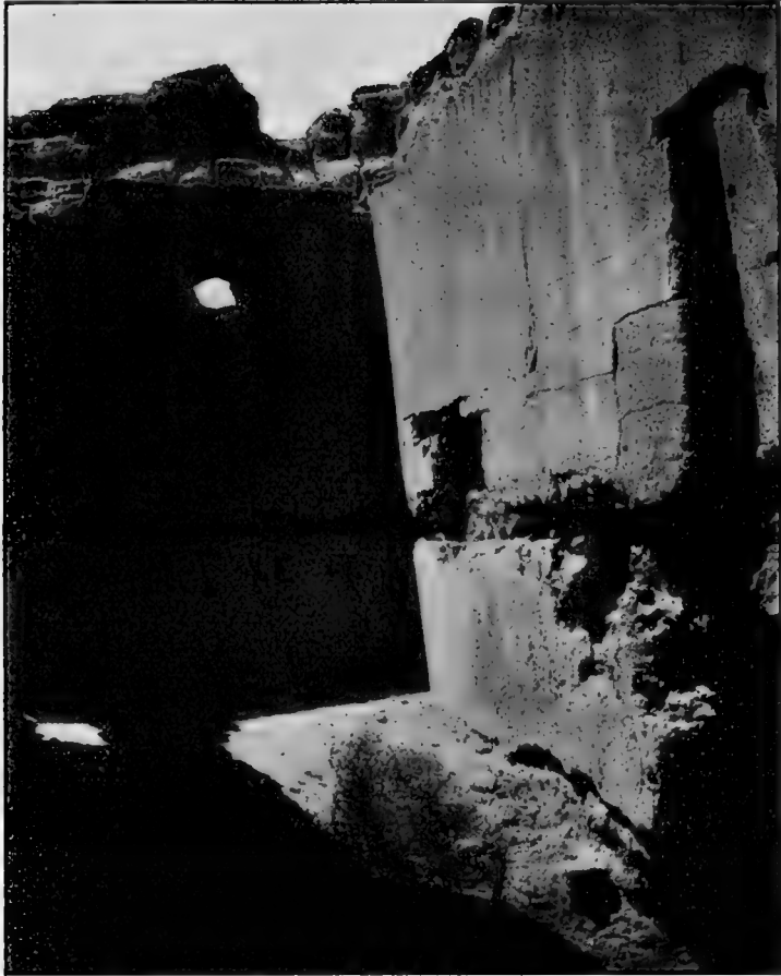
FIG. 9. Interior of north room, looking west.
