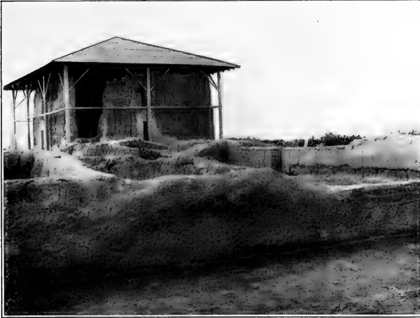
a , NORTH ROOMS
