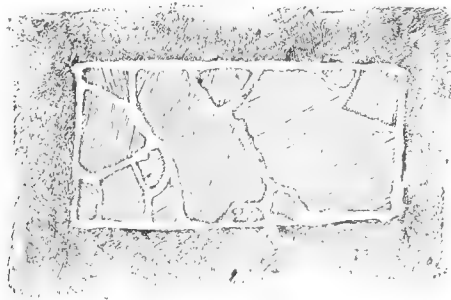
FIG. 90. A Zuñi window glazed with selenite.
