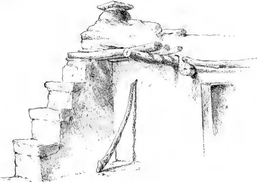
FIG. 49. Stone steps, with platform at chimney, in Oraibi.
