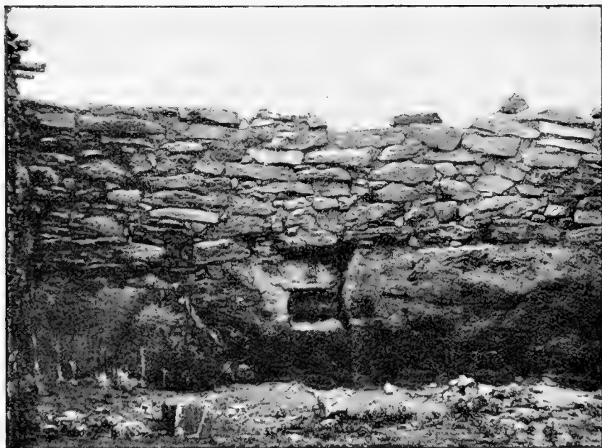
FIG. 35. An unplastered house wall in Ojo Caliente.
