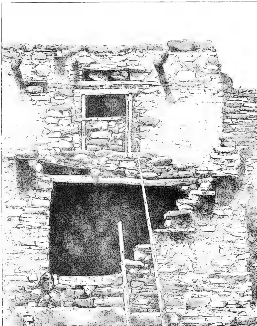
FIG. 79. Rude transoms over Tusayan openings.
