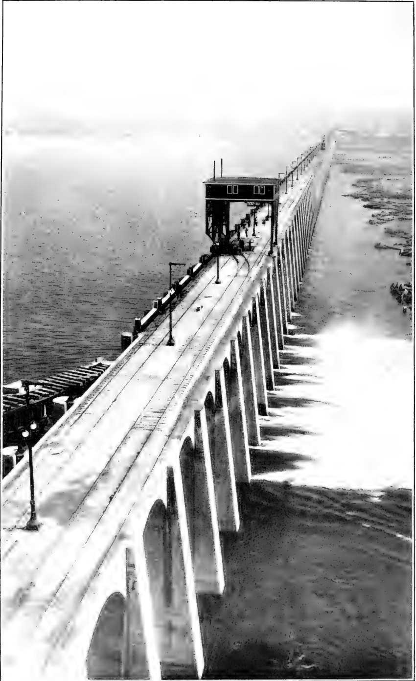
CONDITION BELOW THE DAM WITH SIX SPILLWAYS OPEN. NORMALLY A MUCH GREATER NUMBER OF SPILLWAYS ARE IN USE.
