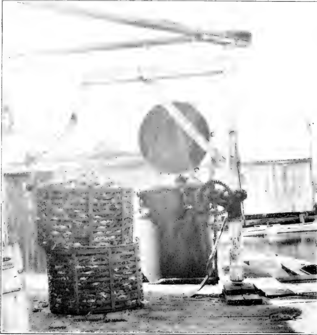
FIG. 1.—IRON COOKER OR "KETTLE," THE USUAL APPARATUS EMPLOYED IN STEAMING HARD CRABS.
