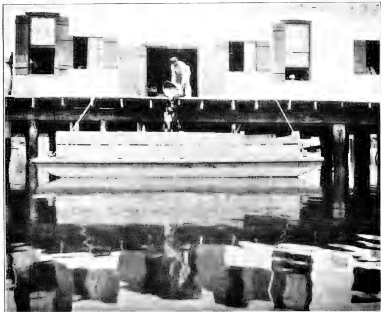
FIG. 2.—EMPTYING "SCRAP" OR WASTE UPON A BARGE TO BE TOWED TO THE FERTILIZER FACTORY.
