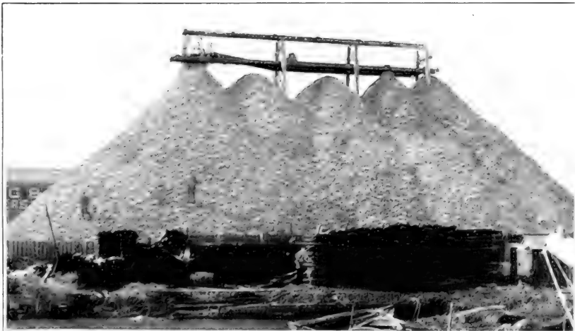
FIG. 2.—SHELL PILE OF A LARGE OYSTER COMPANY, SHOWING CONVEYER FOR CARRYING SHELLS FROM SHUCKING TABLE TO THE PILE.
