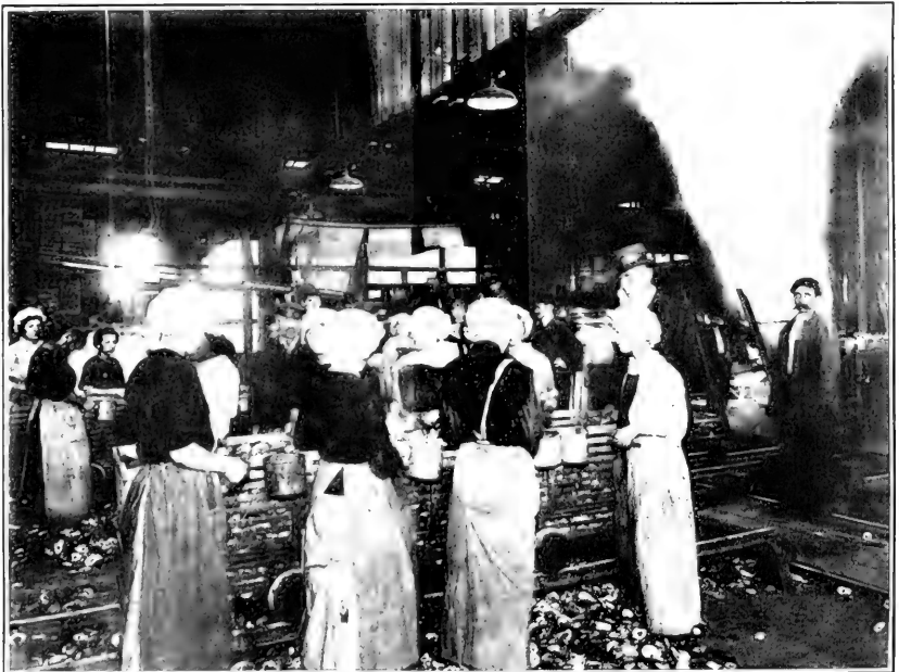
FIG. 2.—INTERIOR OF OYSTER CANNERY; OPENING STEAMED OYSTERS.
