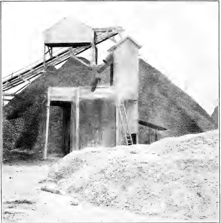
FIG. 1.—KILN FOR BURNING OYSTER SHELLS TO MAKE LIME, SHOWING SHELL HEAP IN BACKGROUND AND PILE OF LIME IN FOREGROUND.
