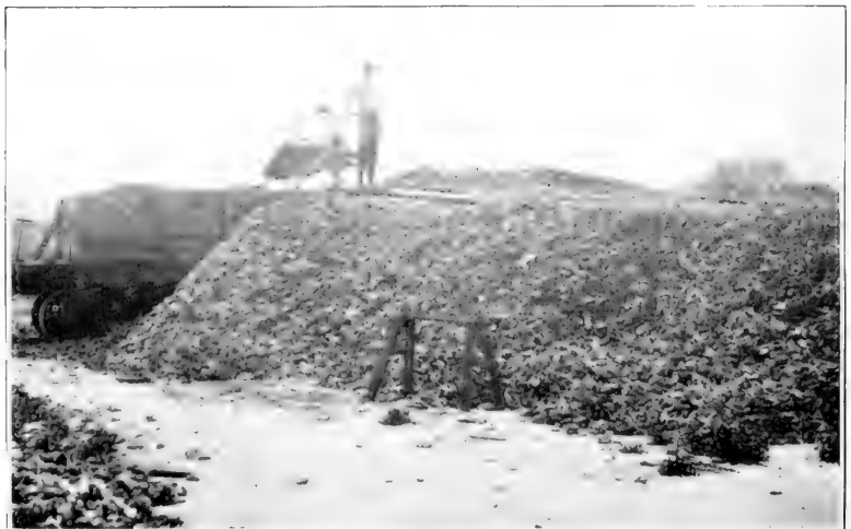
FIG. 2.—LOADING OYSTER SHELLS INTO CAR FOR USE IN BUILDING ROADS.
