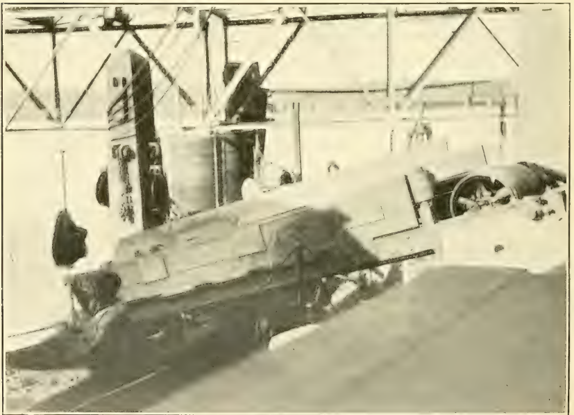
FIG. 2.—UNLOADING OYSTERS FROM THE BOAT AT ONE OF THE LARGE OYSTER HOUSES BY MEANS OF A BELT CONVEYER.
