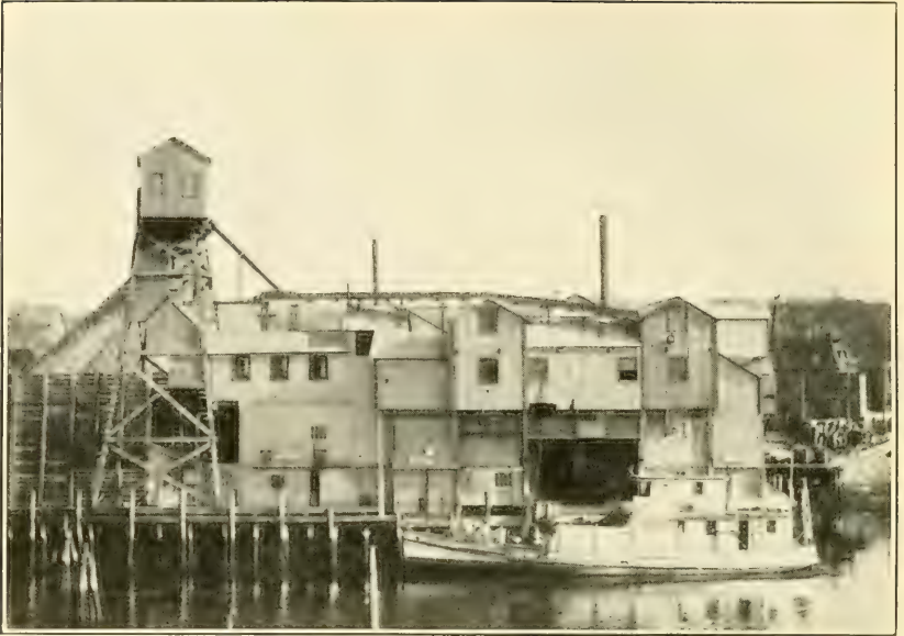
FIG. 1.—LARGE OYSTER HOUSE AT PROVIDENCE, R. I., SHOWING DREDGE BOAT UNLOADING OYSTERS AT RIGHT AND ELEVATOR TO SHELL PILE AT LEFT.
