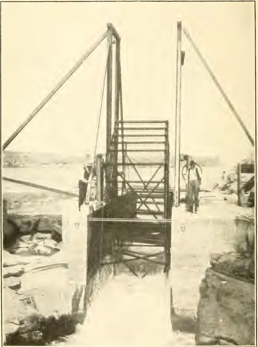
FIG. 25.—A COLUMBIA RIVER STATIONARY FISH WHEEL.
