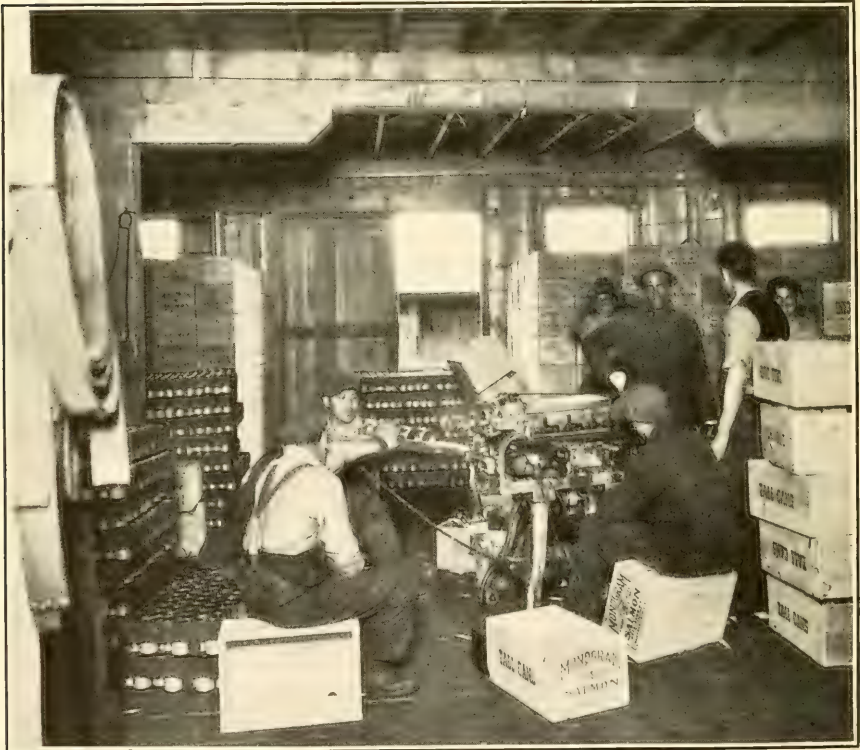
FIG. 34.—SALMON CAN-LABELING MACHINE.
