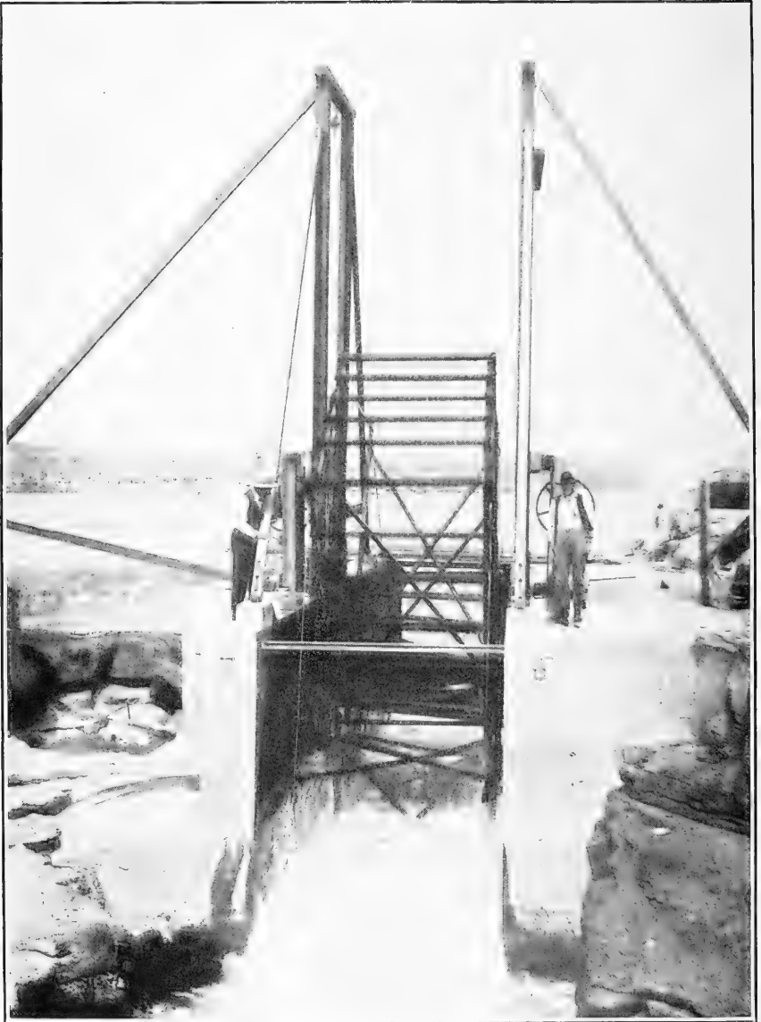
FIG. 25.—A COLUMBIA RIVER STATIONARY FISH WHEEL.
