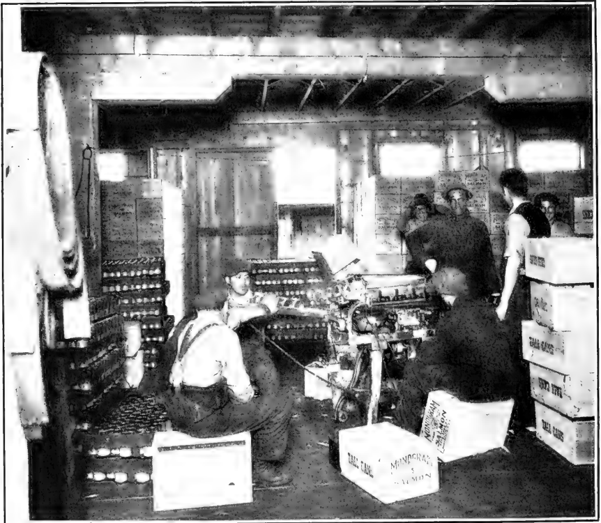
FIG. 34.—SALMON CAN-LABELING MACHINE.
