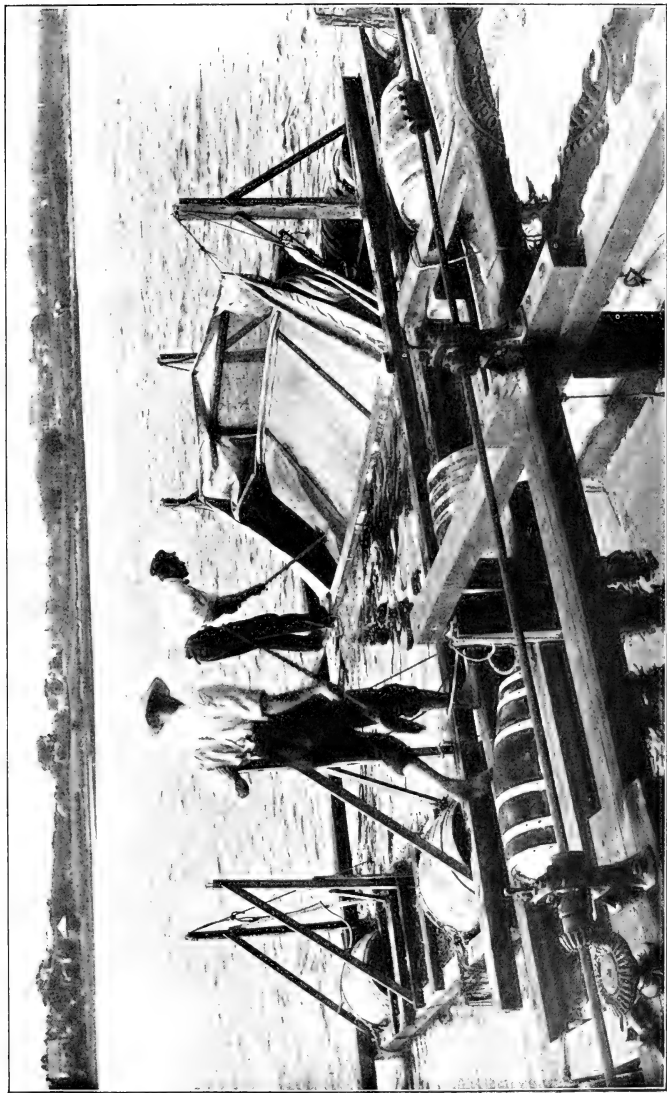
PLATE XIX.—Small float used in cleaning the bags. Shows the method of scrubbing a bag.
