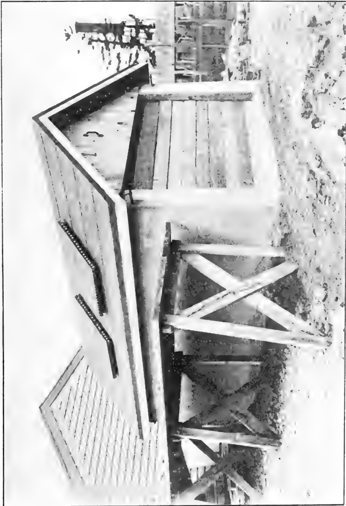
FIG. 36. Photograph of manure shed on poultry plant of Maine Agricultural Experiment Station. Note walk, trap-doors in roof, plank end, and removable gable.
