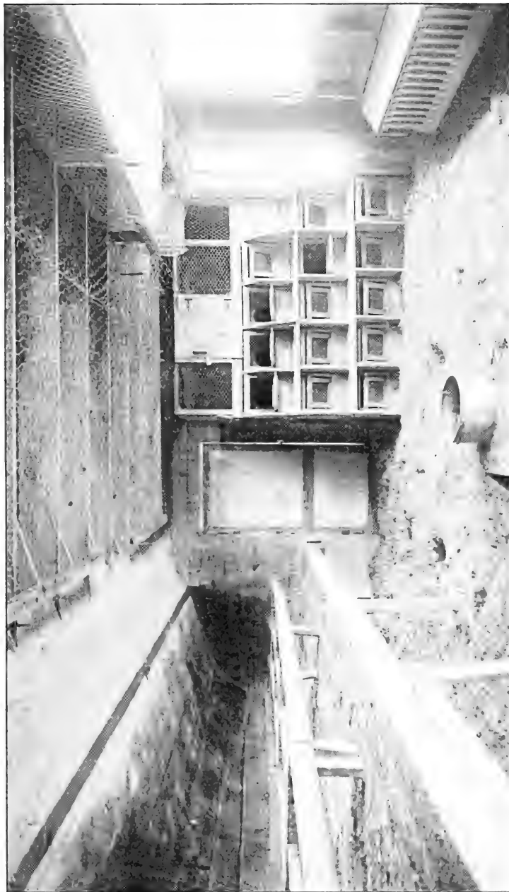
FIG. 16. Interior of curtain front poultry house No. 3.
