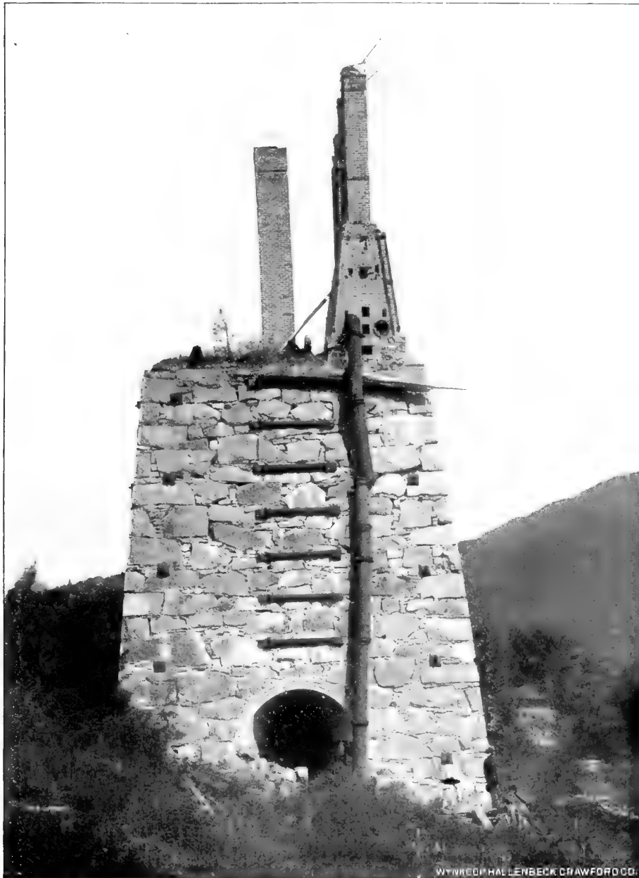
VIEW OF THE BLAST FURNACE AT THE "UPPER WORKS" ON LAKE SANFORD. THIS FURNACE WAS BUILT ABOUT 1852; ITS LINES ARE GIVEN BY A. J. ROSS (TRANS. AMER. INST. MIN. ENG. XXI, PAGE 837). PHOTOGRAPHED BY J. F. KEMP, 1894. SEE PAGE 608.
