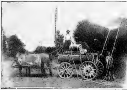
Fig. 100.—Power Sprayer mounted on Wagon.
