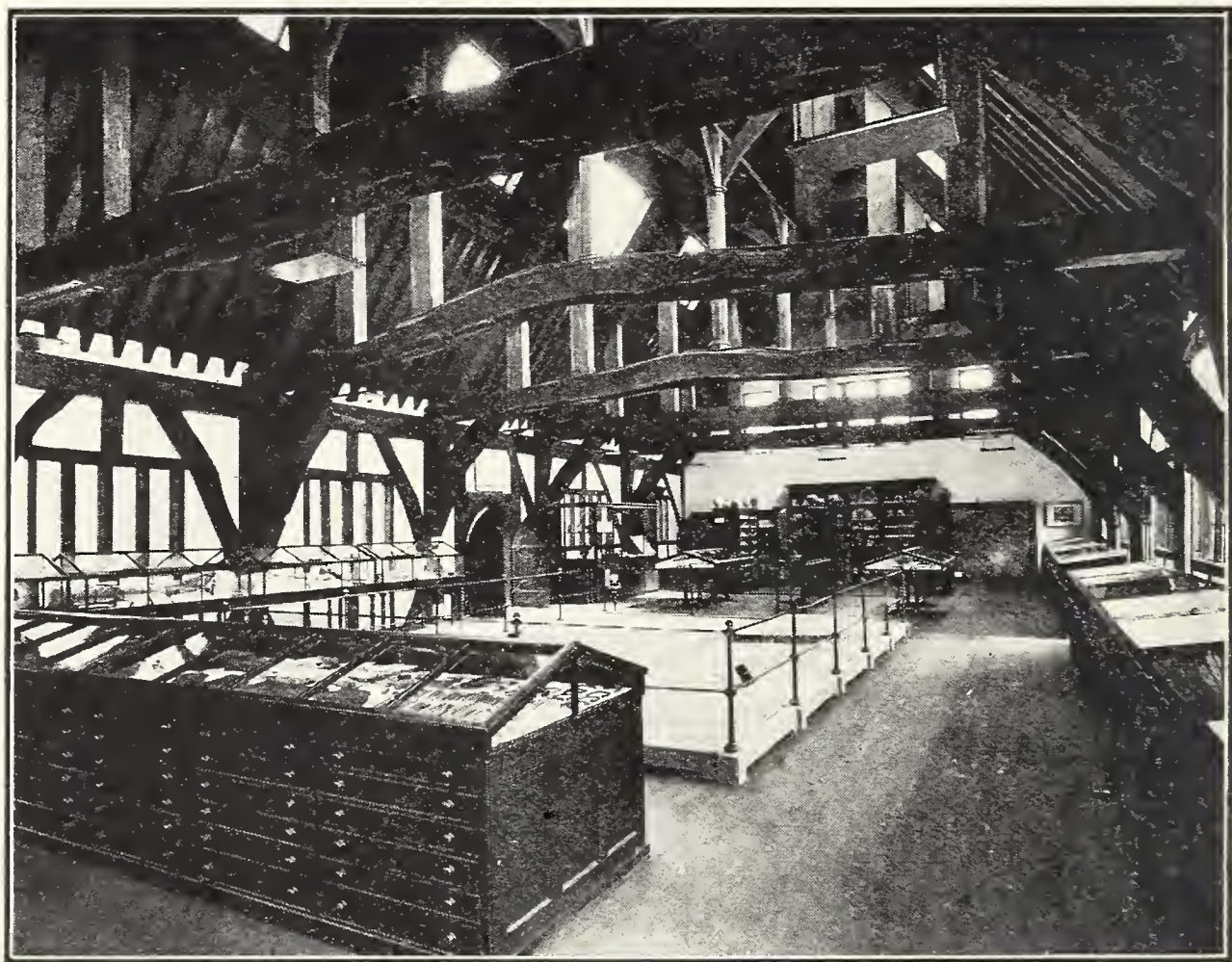
Copyright] THE UPPER ROOM OF THE HOSPITIUM. [Walter Scott
