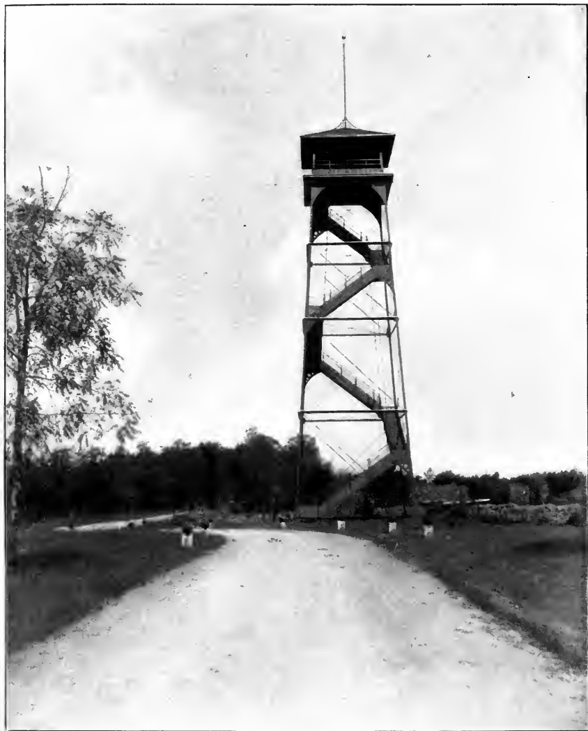
TOWER, CONFEDERATE AVENUE, SECTION 4.
