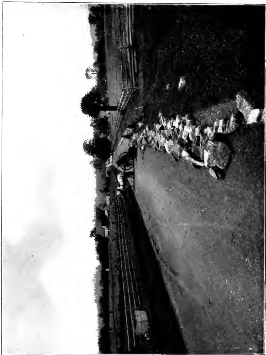
GUTTER PAVING ON UNITED STATES AVENUE.
