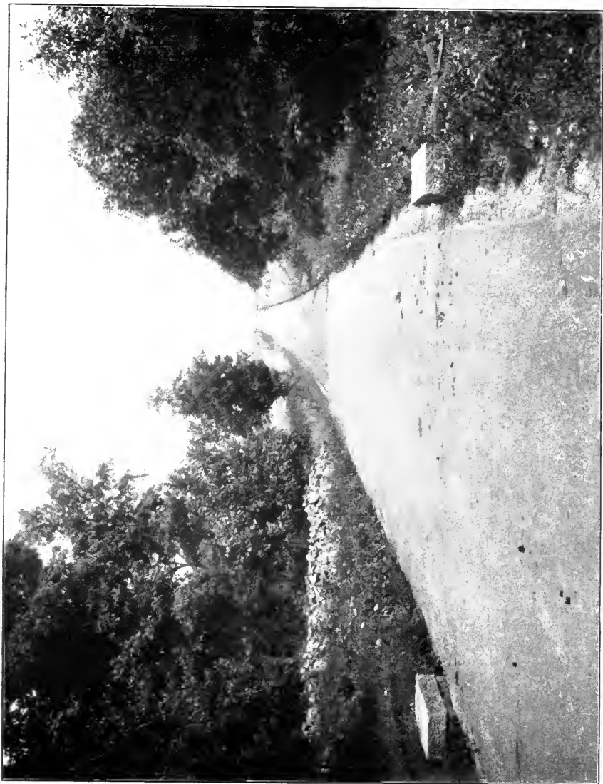
GRADING EAST END OF MEREDITH AVENUE.
