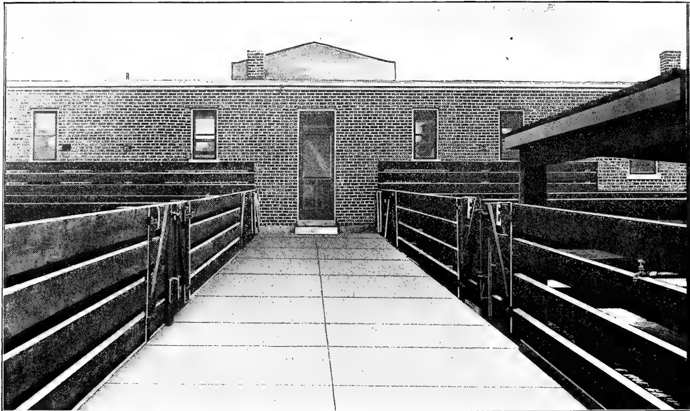
REAR VIEW, Showing Gate Entrance to Pens and Concrete Alley Way.
