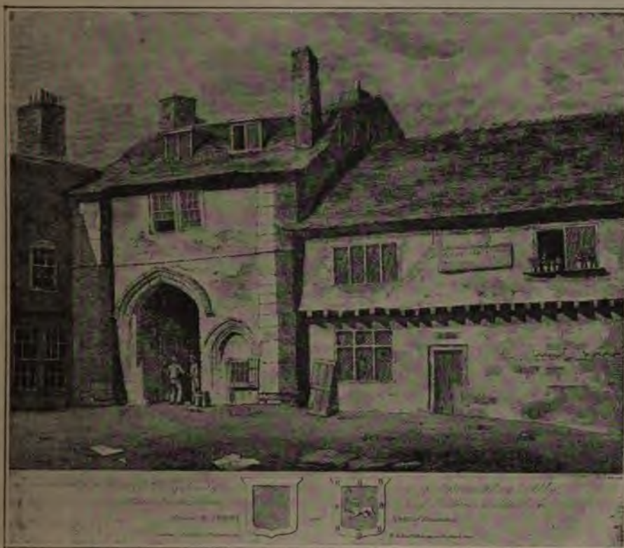
NORTH GATE, BERMONDSEY ABBEY, TAKEN DOWN IN 1805.
