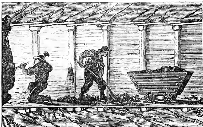
Longitudinal View of Timbered Level.
