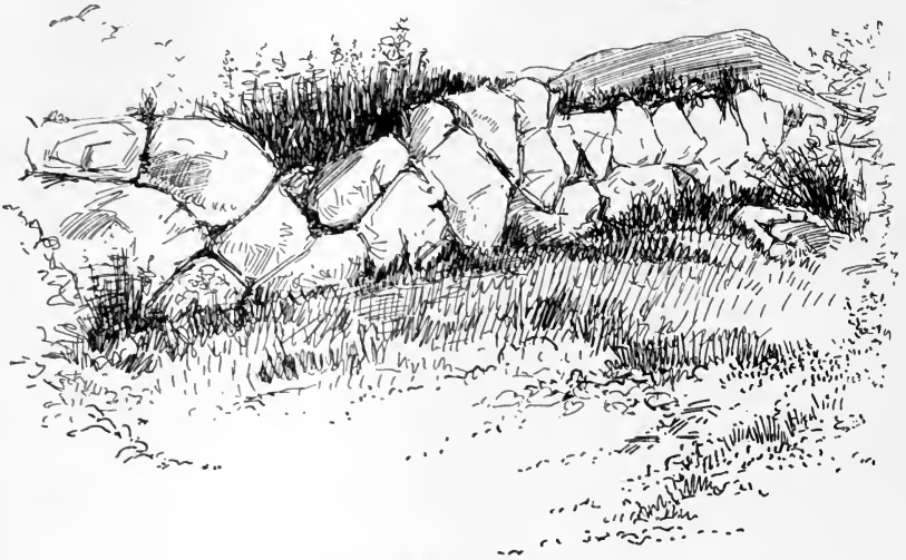
SUSTAINING WALL OF MASONRY.
