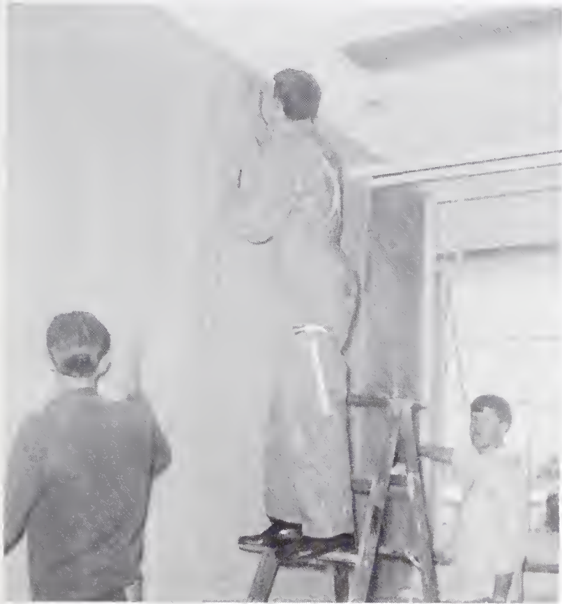
Boys from carpentry class partition Room 2 for guidance offices.
