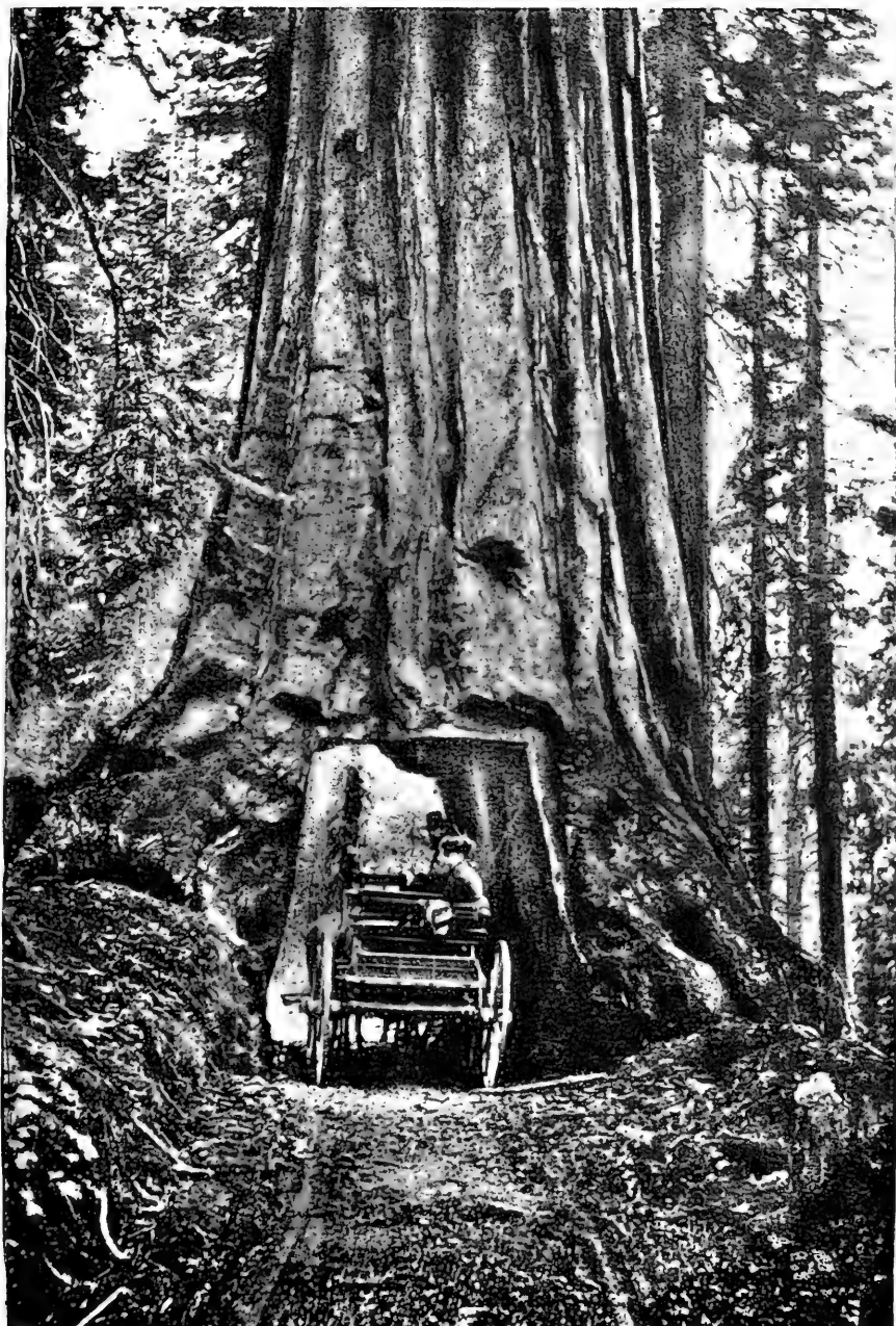
TUNNEL THROUGH "WAWONA." DIAMETER 27 FEET.
