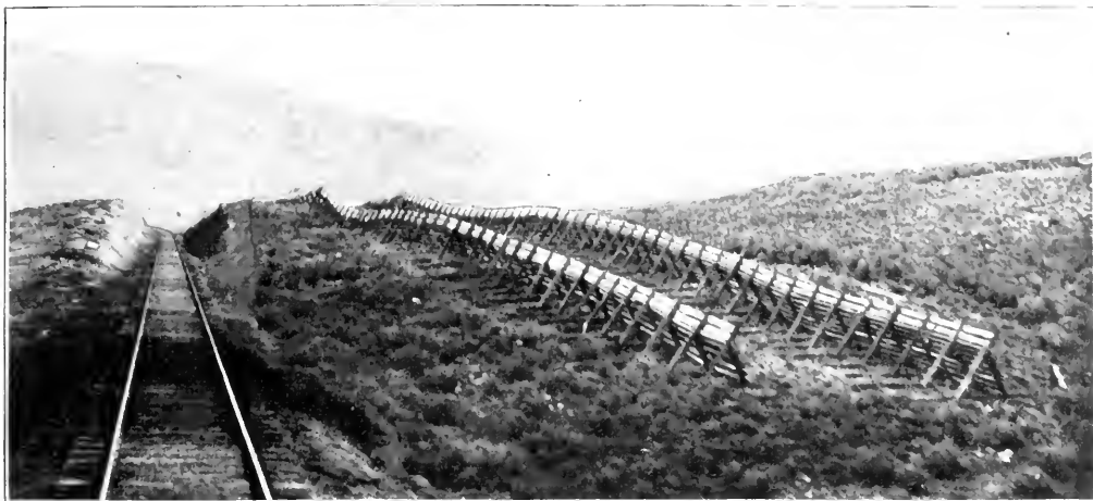
DOUBLE LINES OF SNOW FENCES, SOLDIER SUMMIT, UTAH, ON RIO GRANDE WESTERN RAILWAY.
